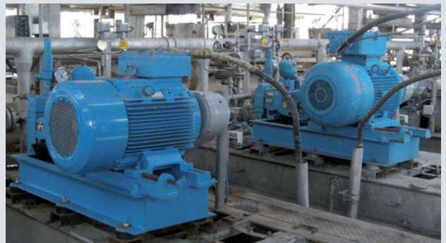
ABEL High Pressure Pump for injection of ethylene in gas drying process
