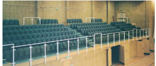
Gymnasium spectator balustrading manufactured from mild steel with a polyester powder coated finish complete with toughened glass infill panels.
