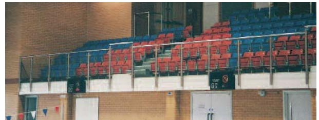
Swimming Pool spectator balustrading manufactured from 316 grade stainless steel complete with toughened glass infill panels.
