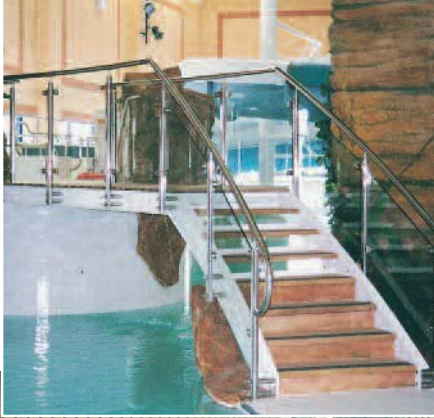
Mild steel bridge, stainless steel toughened glass infill balustrading.
