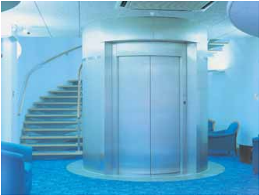
Stainless steel lift shaft cladding.
