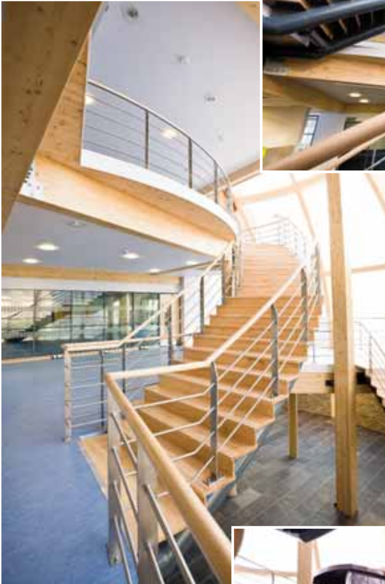
Site: the William Smith Building: a newbuild 4-storey sustainable office facility for the British Geological Survey, Keyworth. Two helical staircases complete with tubular stringers, landings, timber treads and risers, stainless steel balustrading and timber handrail.
