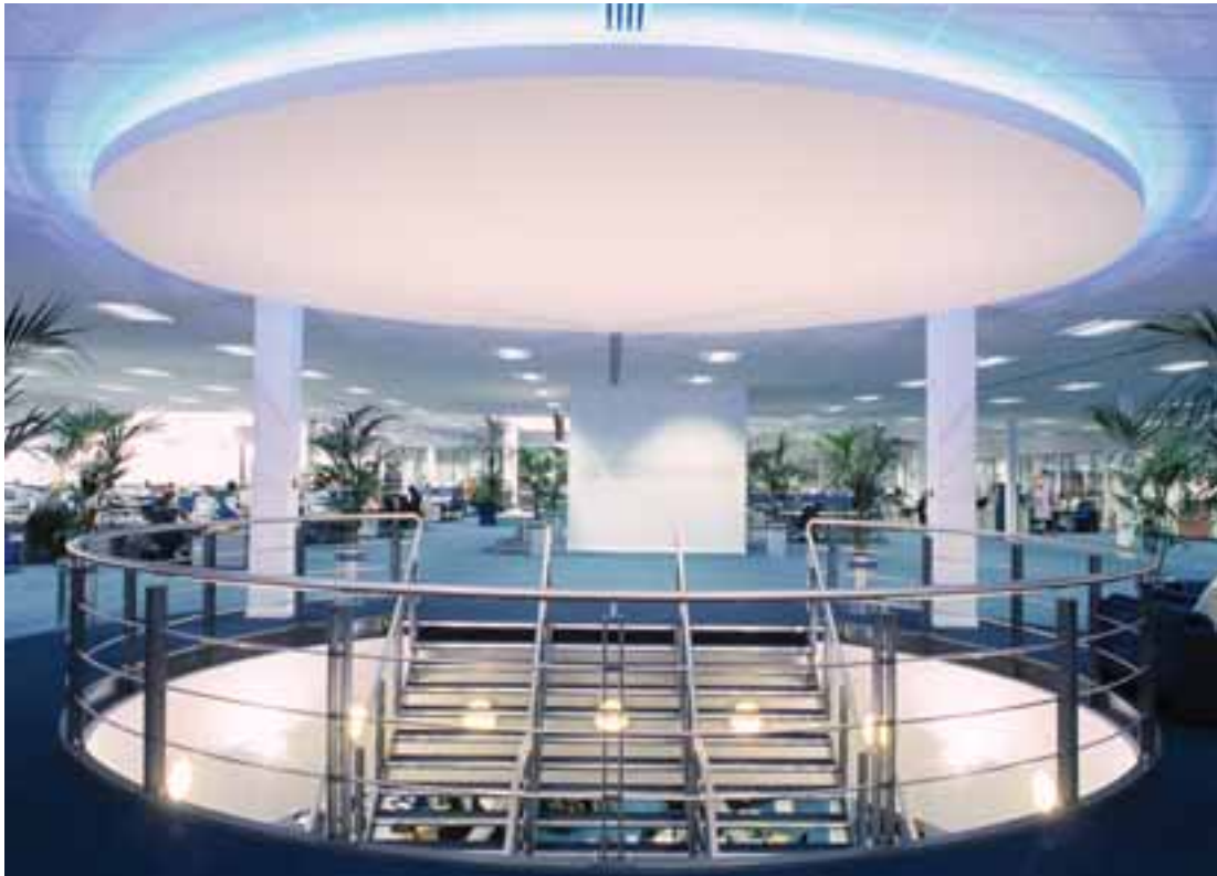
Mild steel polyester coated balusters complete with stainless steel rod infills and top rail.
