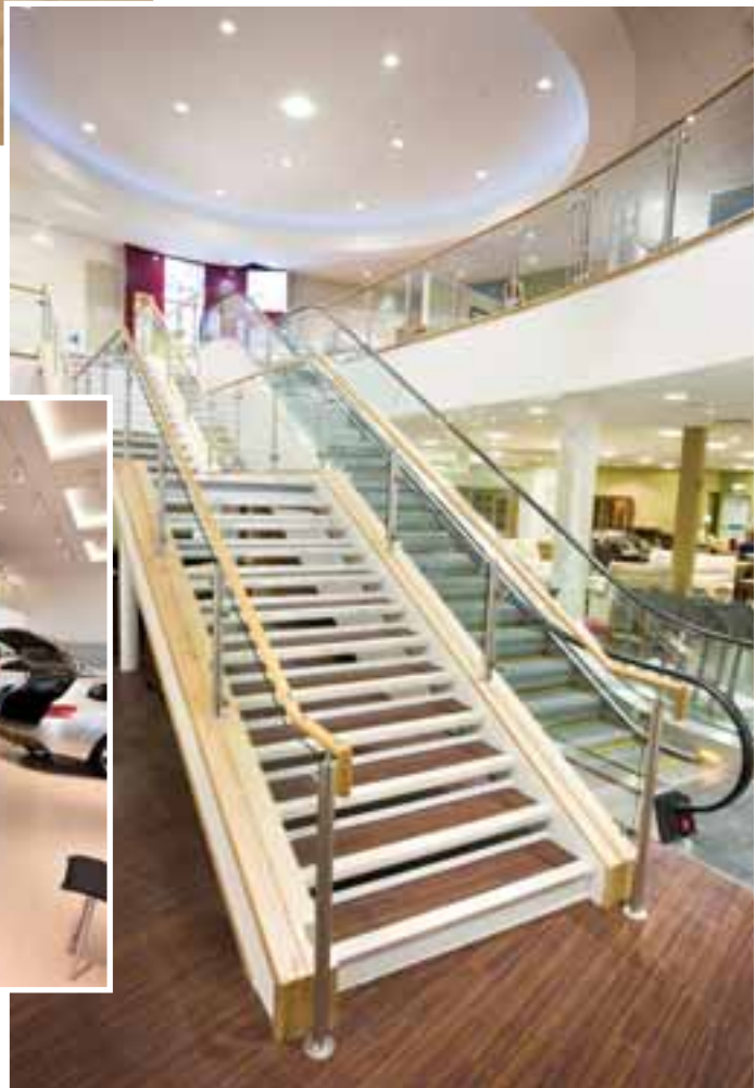
Feature stair complete with glass infilled stainless steel balustrade, solid oak capping and top rail
