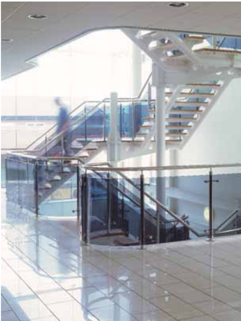
Polyester powder coated staircase complete with glass infill balustrade. Project: Searchlight, Manchester
