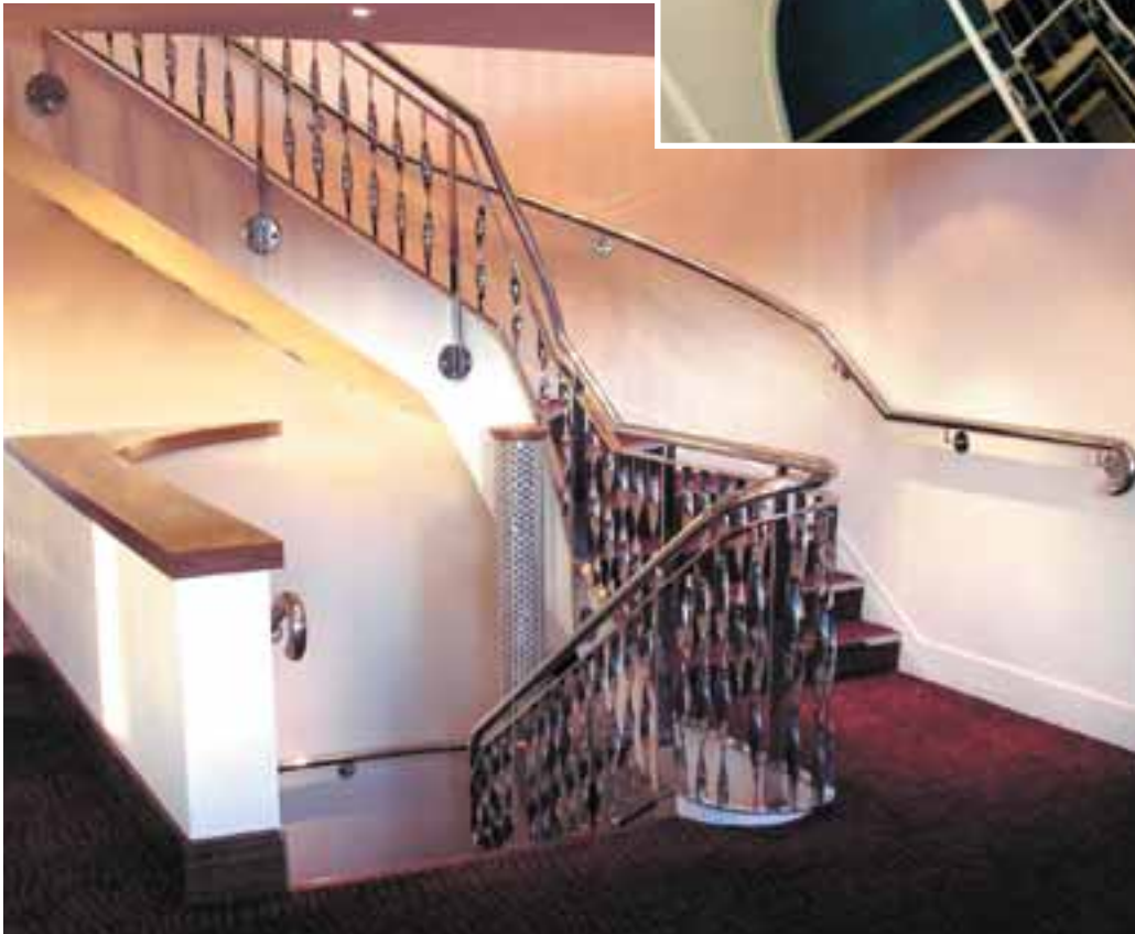
Stainless steel balustrading complete with a flat bar twist infill. Project: Nightclub, London.
