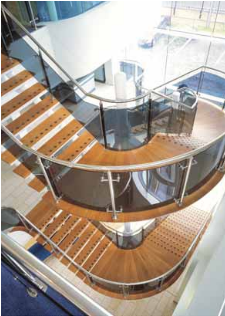
Curved glass complements the balustrading on this feature staircase at Searchlight Electric in Manchester.
