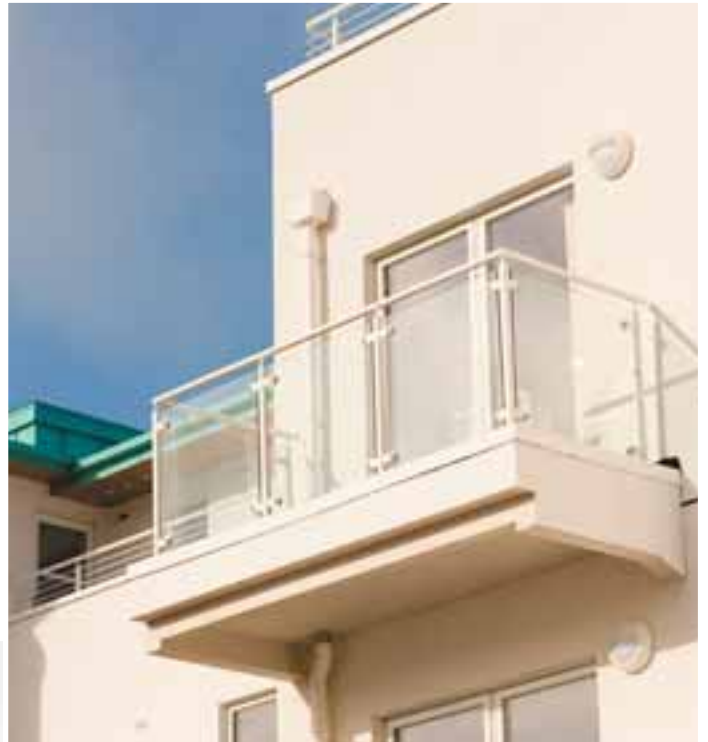
Polyester powder coated glass infill balcony balustrading to luxury apartments, Holyhead Marina.
