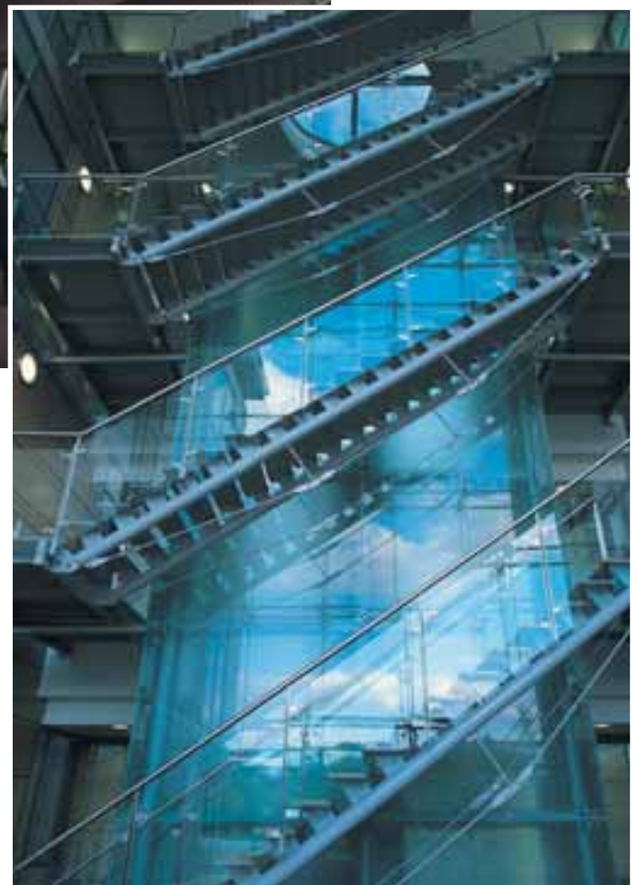
Four flight staircase complete with glass balustrading and timber treads and landings.
