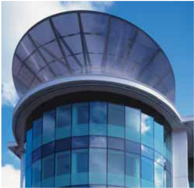
Structural steel framework with a perforated sheet cladding form an impressive feature to this office block roof.
