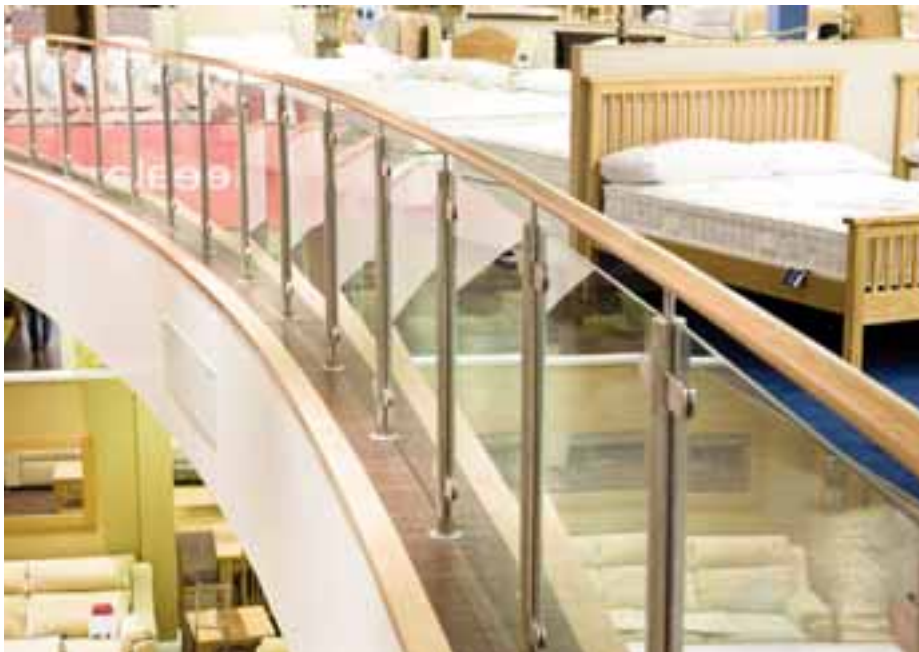
Curved atrium balustrading complete with timber top rail.
