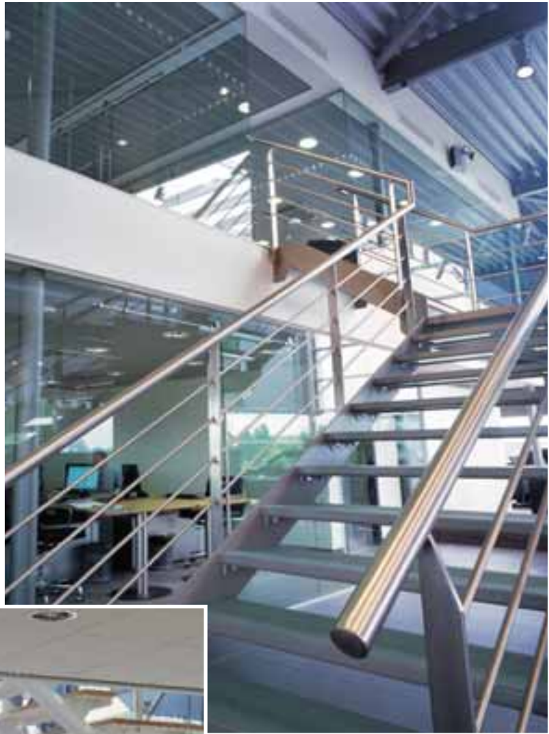
The glass infilled tray type treads complement this staircase.
