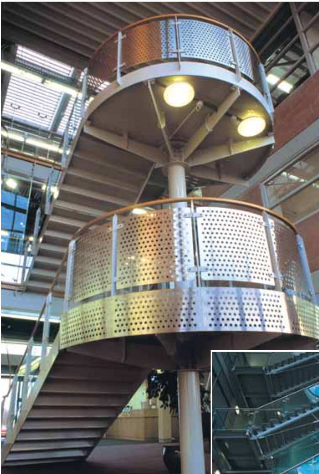
Mild steel staircase landings, support column complete with glass and stainless steel perforated sheet infilled balustrading and timber top rail.
