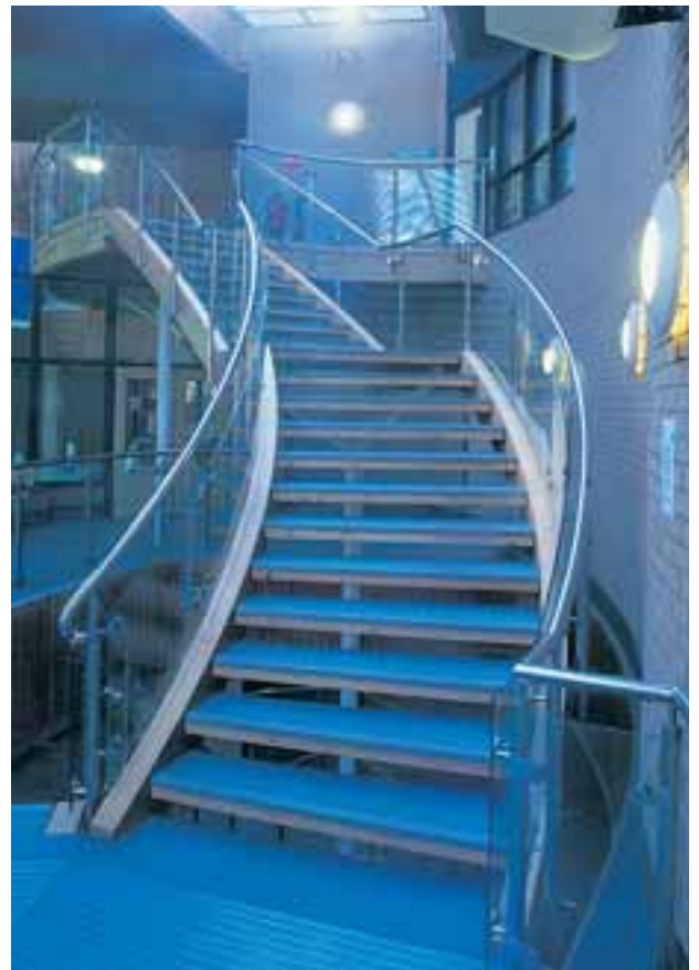
Stainless steel curved balustrading with curved toughened glass infills complete this staircase perfectly at The Quays Swimming & Diving Centre in Southampton.
