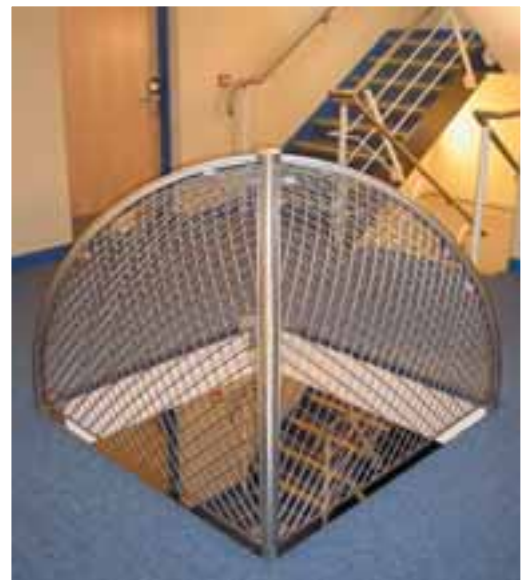
Stainless steel light-well dome complete with 6mm fabricated mesh infill.
