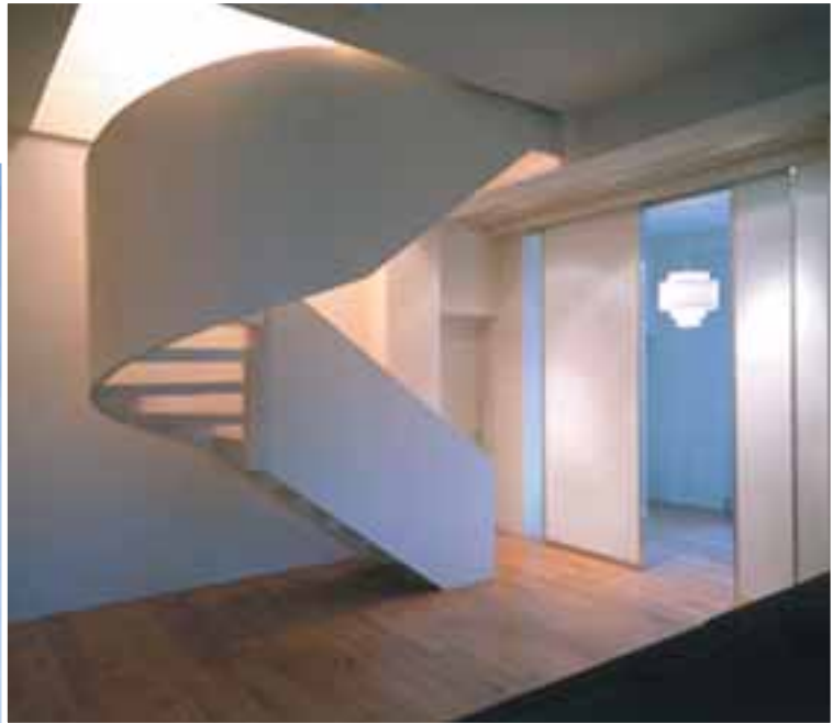
Mild steel staircase complete mild steel sheet-clad balustrade for Quinn Architects.
