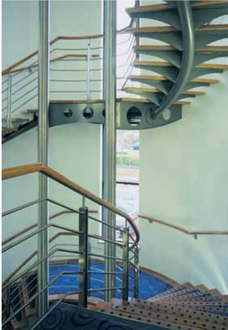
Mild steel polyester powder coated helical staircase and stainless steel balustrading complete with stainless steel support columns, timber treads and top rail. Situated in the prestigious offices of a surgical instruments manufacturer.
