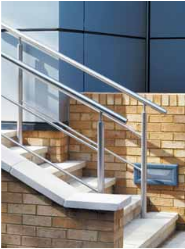
Stainless steel balustrade to external steps.
