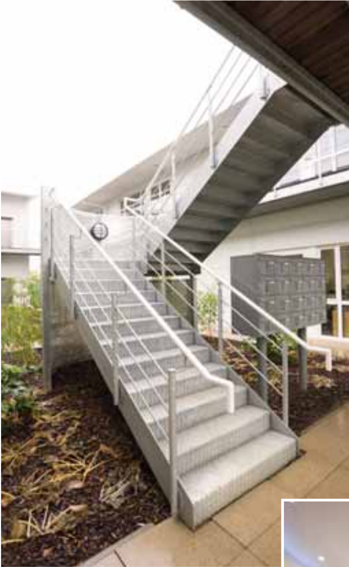
Galvanised mild steel external staircase, complete with galvanised balustrade and handrail and semi-circular perforated aluminium infill panels
