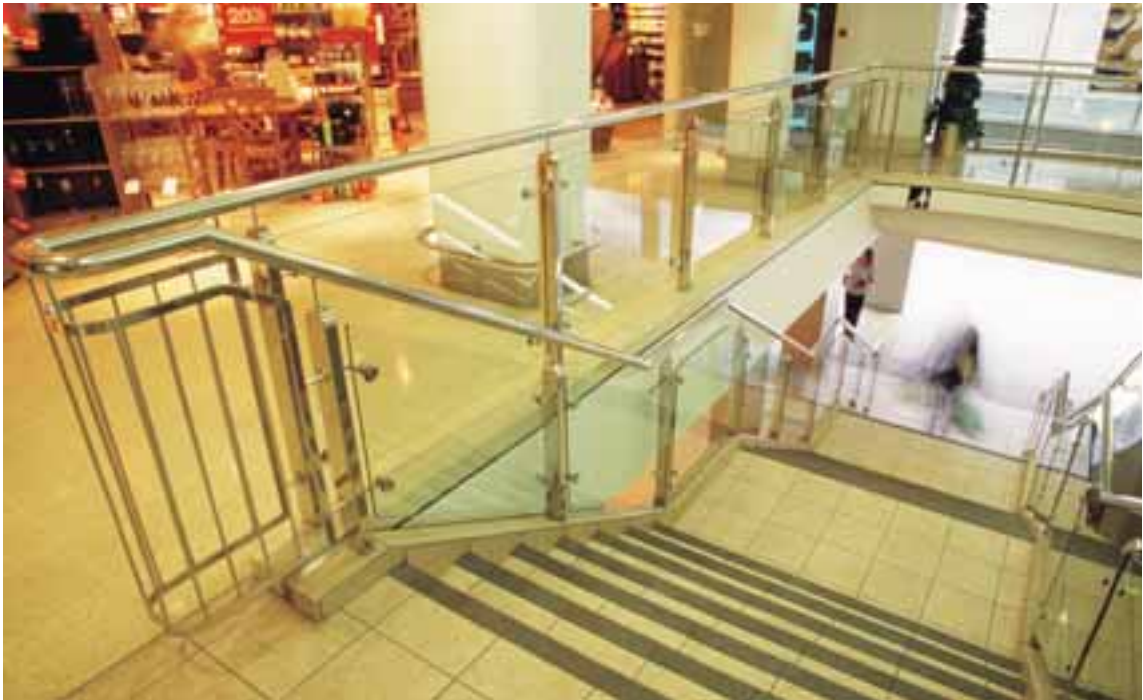
Stainless steel glass infilled balustrading to shopping centre stairwell and balcony.
