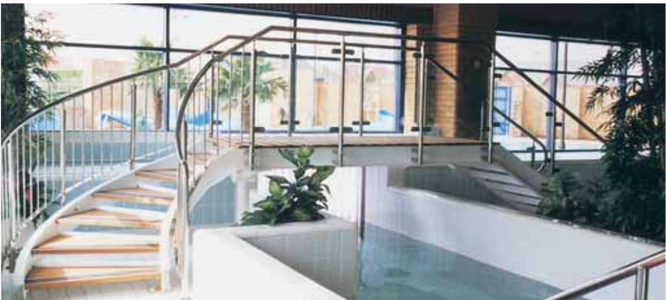
Mild steel bridge, stainless steel balustrading complete with toughened glass and stainless rod infills. Designed by M & G Olympic Products Design & Development Department.
