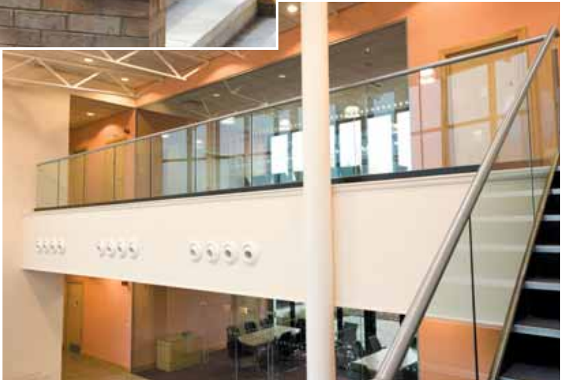
Structural glass balustrade with stainless steel top rail.
