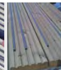
Q-Grip® Strips fitted into Q-Deck® York
