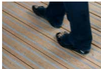
Fig (ii) Boards parallel to pedestrian traffic.
