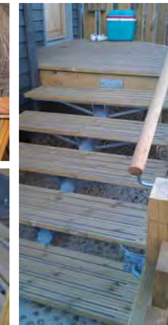
Q-Grip® Strips in Q-Deck® Lunawood finished with Aquadecks Teak (image top left).
