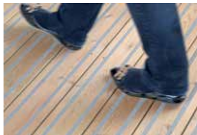
Fig (i) Boards placed at right angles to pedestrian traffic.
