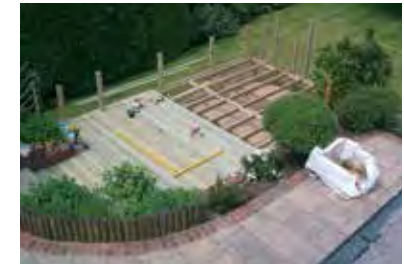
....fixing the deckboards throughout the deck....
