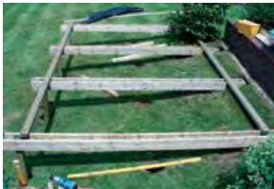
....building the support beams....
