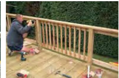
....fixing the balustrades....
