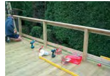
....fixing the handrails and base rails....
