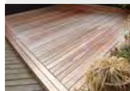
Q-Deck ® Lyptus showing early signs of weathering.
