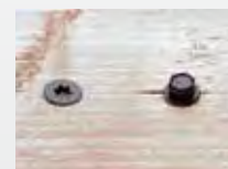
Timber-Tite countersunk versus proud hex head.
