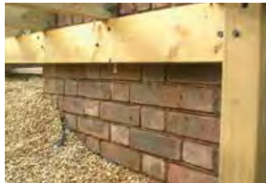
....ledger board fixed to existing wall....
