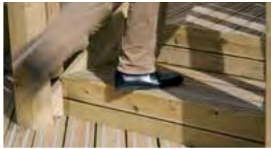
Step frame set on compacted hardcore and weed barrier.
