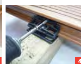
Central screw, expansion left and right.
