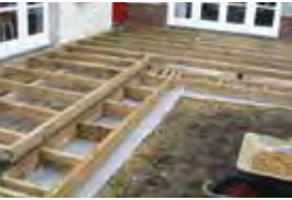
Step frame set on compacted hardcore and weed barrier.
