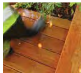
Q-Deck ® Garapa being cleaned with Net-Trol.
