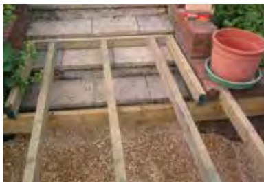
....ledger board fixed to existing steps....
