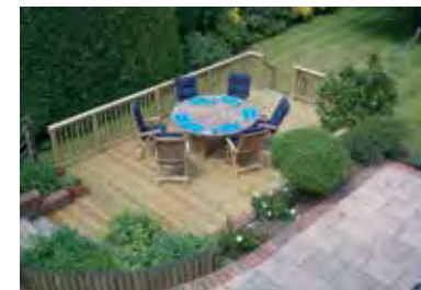
....the completed deck....
