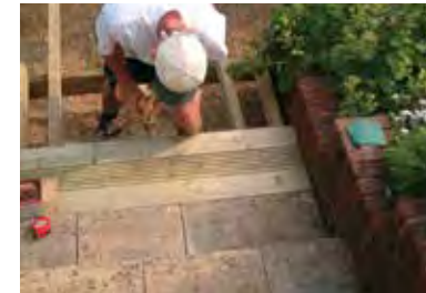
....fixing the first deckboards....
