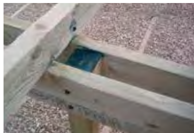
....joist fixed over the beams....
