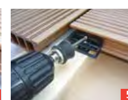
Screw at end, expansion all to right.
