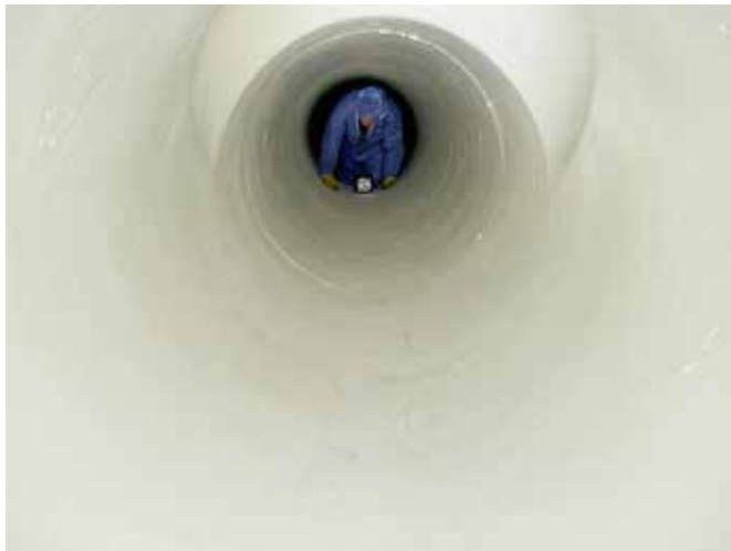
Rehabilitation of a GRP pipe used as part of an air-conditioning system
