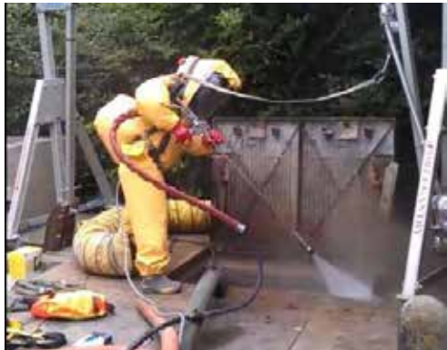
Saturation blasting a concrete pumping chamber
