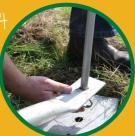
Lay the strut on the plate, hook tension wire through pin & drive in
