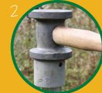
Erect end strainer/corners by digging or driving in manually or mechanically
