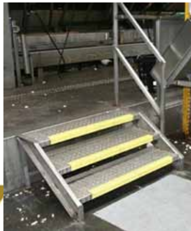
Nosings are standard 55mm x 55mm
