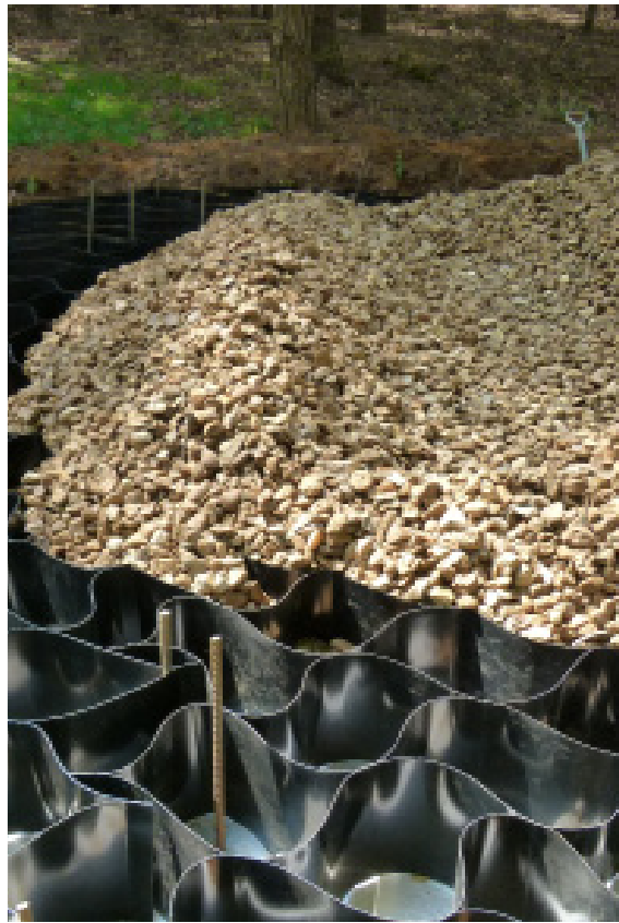
Abweb opened and infilled with 'no-fines' stone fill
