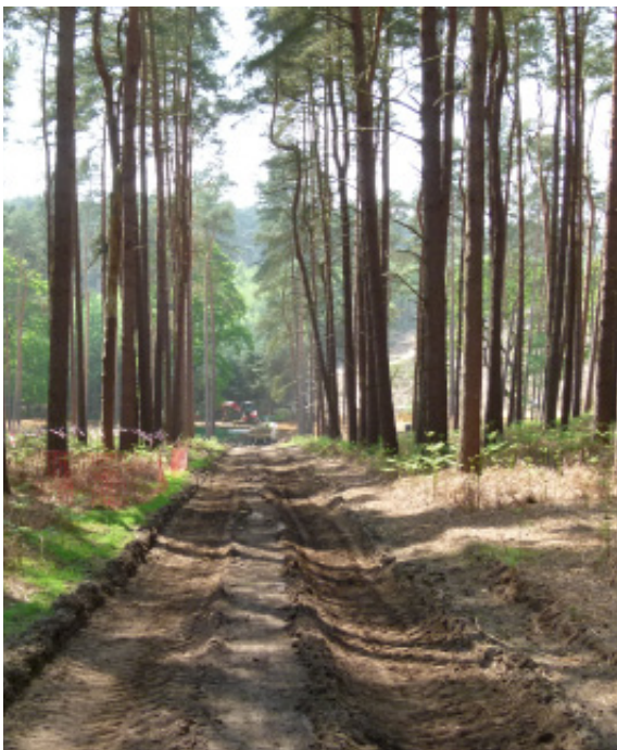
Access track prior to installation of Abweb system
