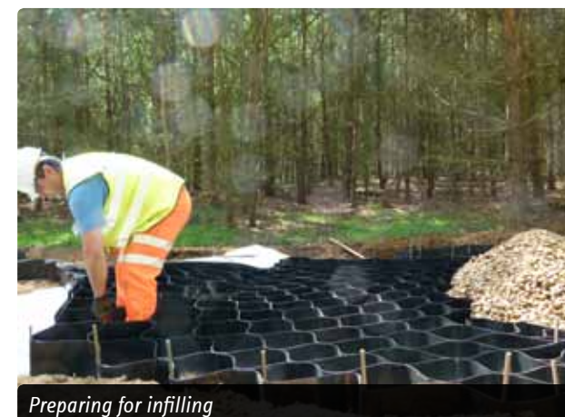
Inserting temporary pins to hold cell panel open
