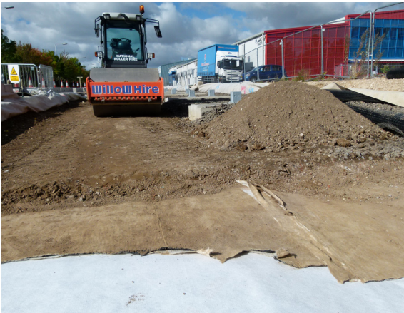
Pozidrain being covered over prior to installation of precast track sections
