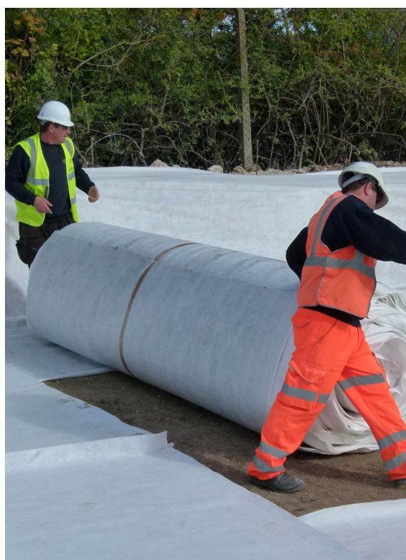
Installing Pozidrain Geocomposite drain at formation level
