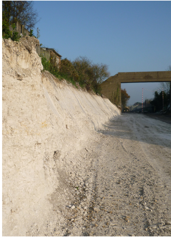
Embankments prior to Erosaweb installation
