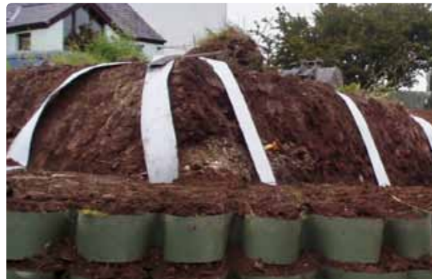
Fildrain installed as drainage strips behind Webwall installation
