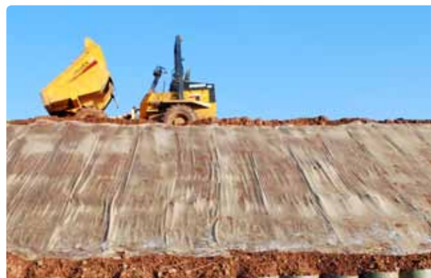
Erosamat Type 1 installed on upper slope of Webwall installation
