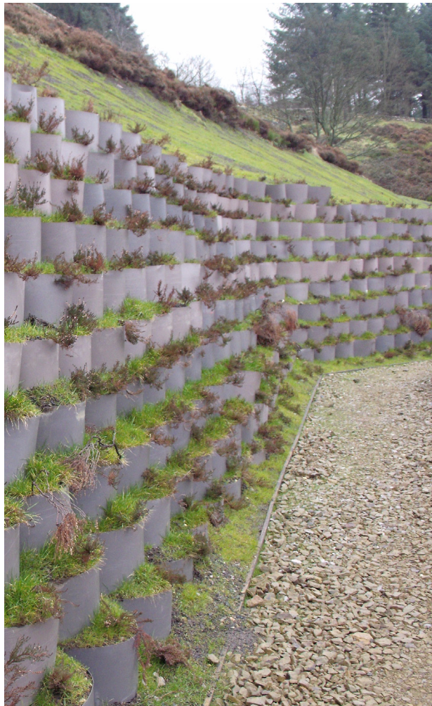
Embankment post installation
