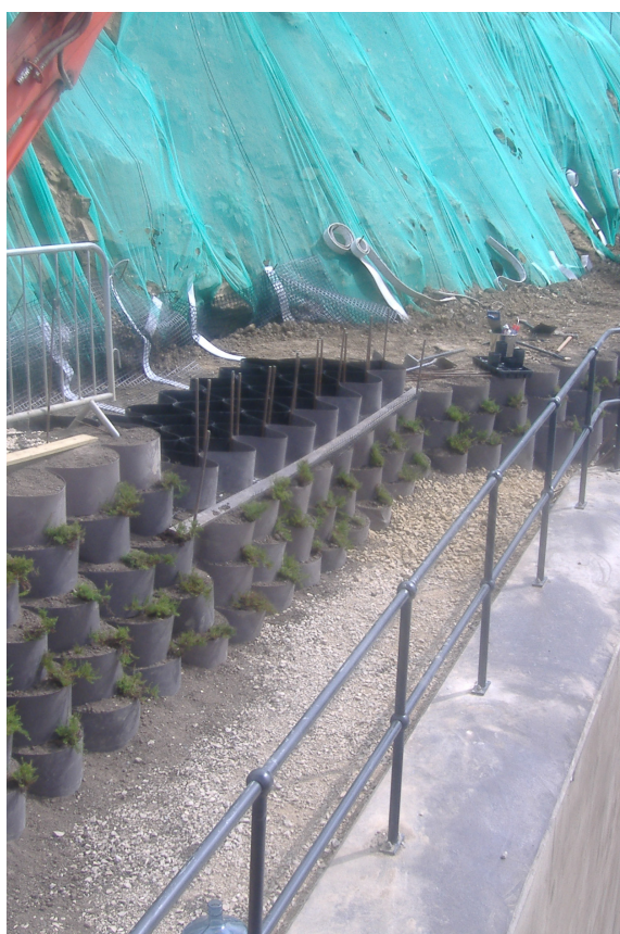
Webwall structure mid-installation
