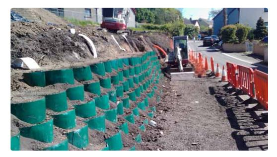
of the embankment. This negated the need and cost of importing additional materials to site. Upon completion the newly built wall was replanted with vegetation and the structure was allowed to naturally restore its green appearance. This was in keeping with the surrounding environment.
