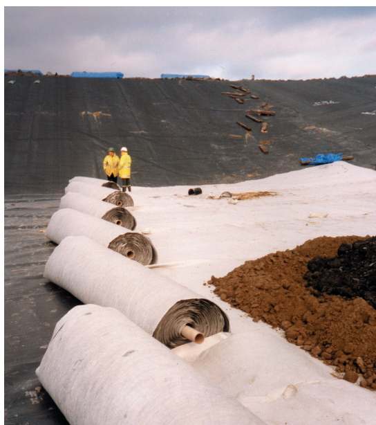
Large Pozidrain rolls allow rapid coverage
