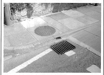
The Kinghurst bypass kerb maintains channel continuity when kerb to kerb road humps and speed tables are built.
