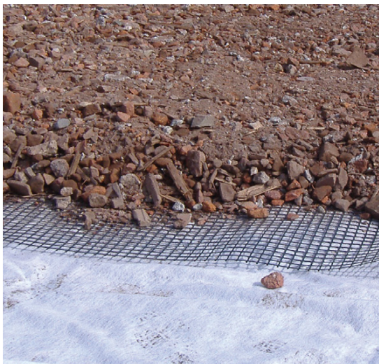
Terrex overlaid with Abgrid and then hardcore fill to form sub-base
