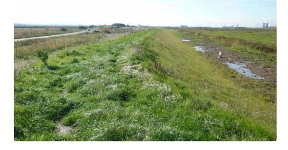
The Greatham flood alleviation scheme comprises the raising of and improvements to existing flood defences originally constructed in the mid to late 1800's by the formation of embankments and bunds.
