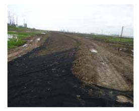
The works include the construction of a new embankment alongside the A178. The embankments are 2.5m high with 1 in 3.5m to 1 in 4m side slopes dependent on ground conditions. The width across the top of the embankment is approximately 3m.
