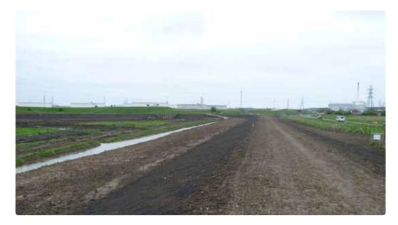
Following installation of the Erosamat and top soil the area was conventionally seeded to allow vegetation to develop.
