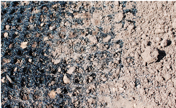
Erosamat Type 3 with imported top soil laid on. Note the soil particles filling the Erosamat Type 3 matrix
