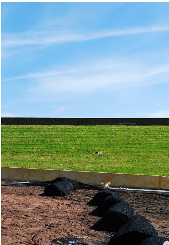
Erosamat Type 3 rolls positioned prior to unrolling
