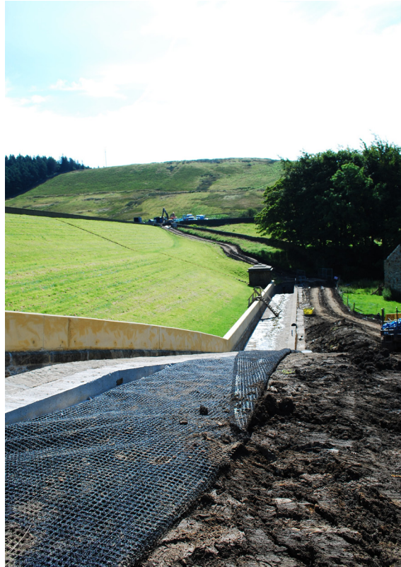
Erosamat Type 3 unrolled and place down embankment
