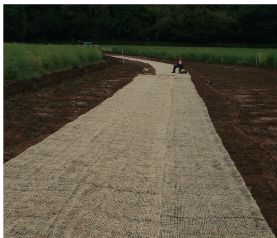
Erosamat laid prior to seeding
