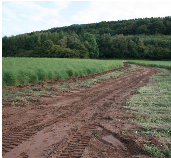
Preparing the water way prior to laying Erosamat
