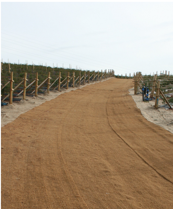
Erosamat Type 2: Laid in Blueberry Field prior to seeding
