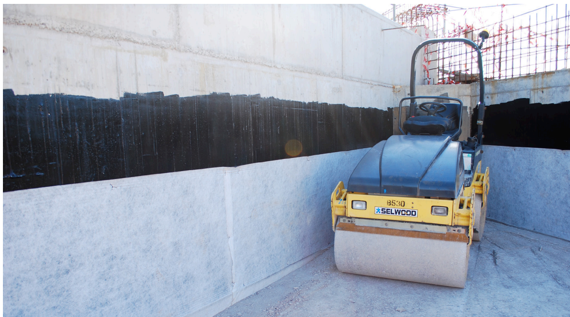
Deckdrain positioned against RC concrete wall with backfill material being compacted.
