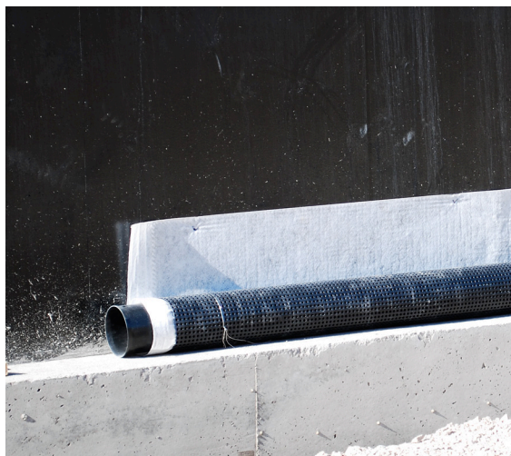
Deckdrain against liquid applied structural waterproofing
