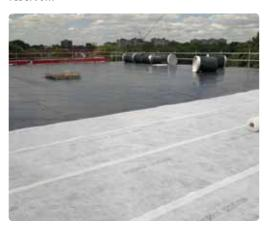
As with all underground reservoirs drainage is a major consideration to ensure longevity of the construction. From the start of the project the design team were keen to adopt innovative technologies and chose Deckdrain as their drainage solution.
