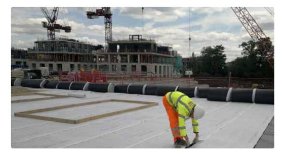
In total 8,000m<sup>2</sup> of Deckdrain has been installed against both the reservoir walls and roof providing drainage and protection.
