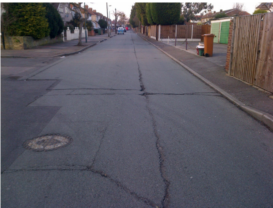
Fen Grove before rehabilitation works
