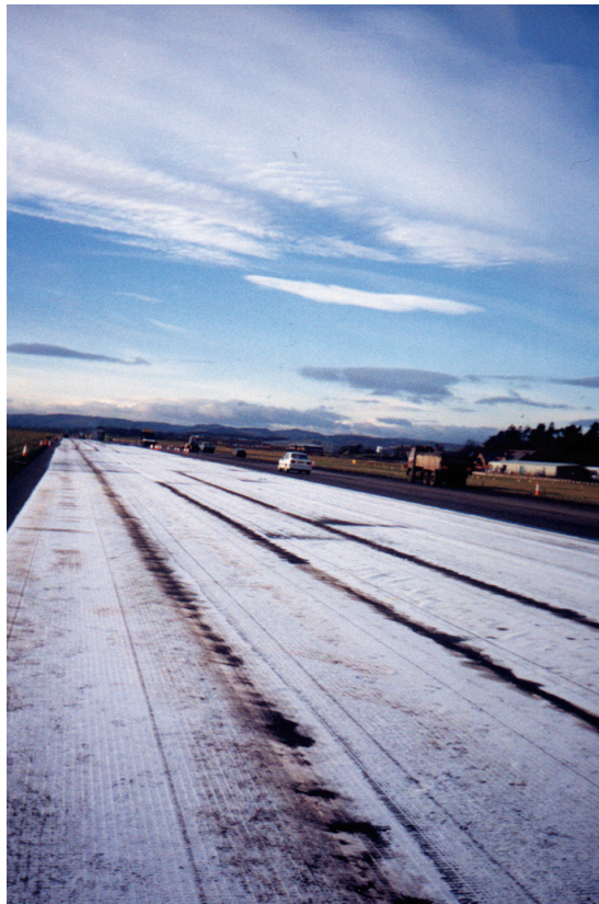
Rotaflex in-situ prior to application of asphalt overlay.
