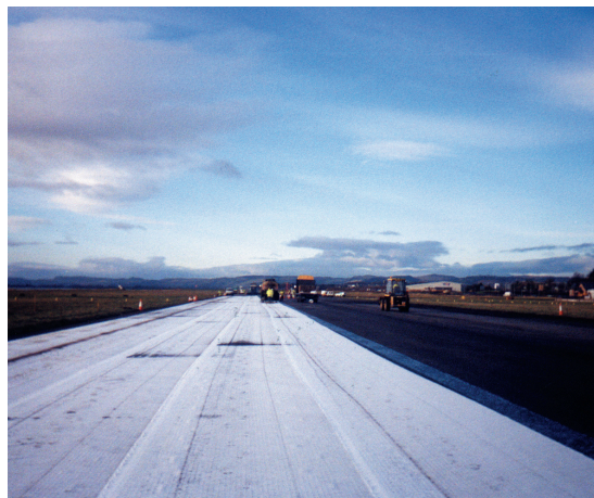
Asphalt reinforcement prior to asphalt overlay
