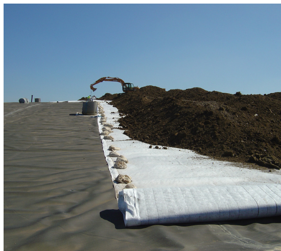
Pozidrain positioned over capping geomembrane with soil backfill placed on top.
