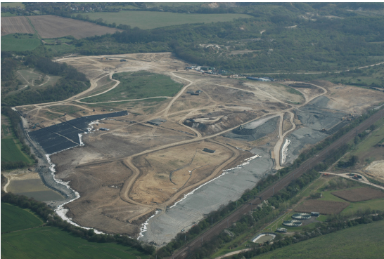
White areas in front of soil backfill show Pozidrain drainage layer. (Photo courtesy of Bedfordshire County Council)
