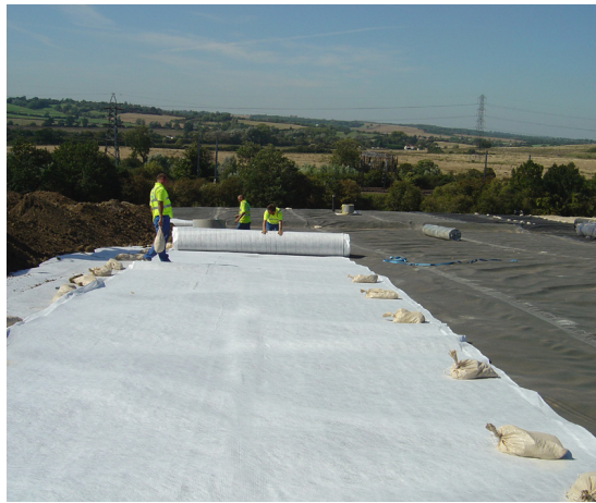
Pozidrain being unrolled prior to backfill being placed.
