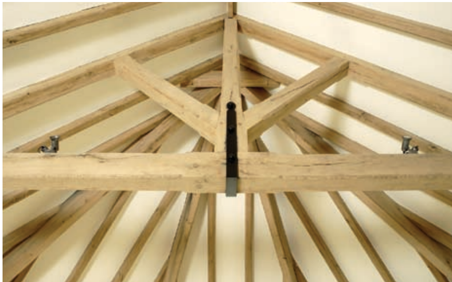
Oak truss, Shropshire
