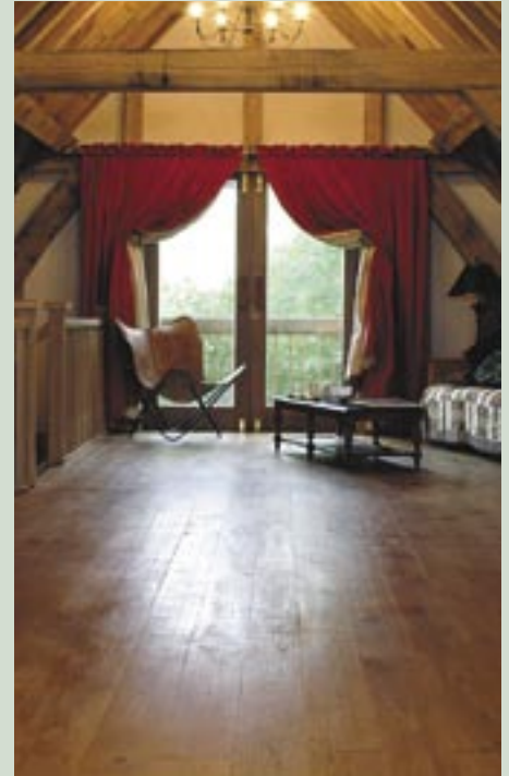
5-metre long flooring for uninterrupted lengths to replicate old oak flooring.
