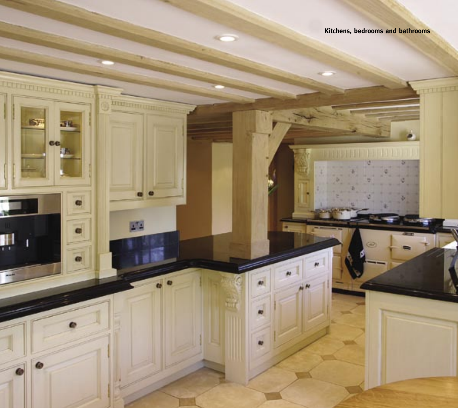
The kitchen above was part of an extension to a 16th century oak-framed Wealden Hall house. The false ceiling beams are made from Orlestone air-dried oak, and the structural steel post was enclosed in a hollowed-out oak beam
