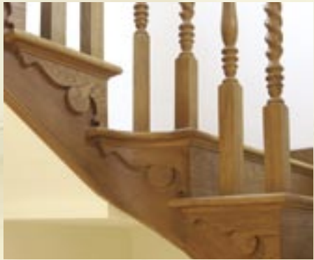
The oak staircase shown on this page has a curved outer cut string on the quarter landing. It also features alternating spindle designs and carved newel posts. Orlestone Oak fitted 12 internal oak doors at this property and all interior oak was French polished on site.
