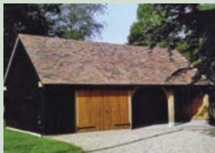
Three-and-a-half bay garage/workshop
