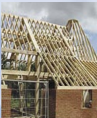
Softwood was used for the rafters on the oast house roof.
