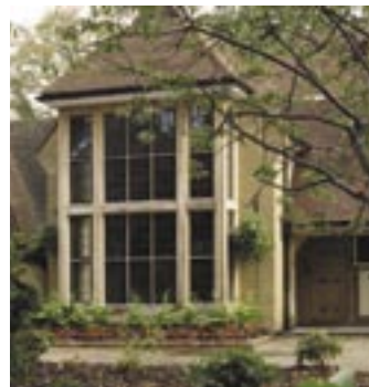
Gallery window This solid oak frame was constructed from air-dried oak beams. Orlestone Oak joinery and timber products were specified as part of a major refurbishment of a large family property.
