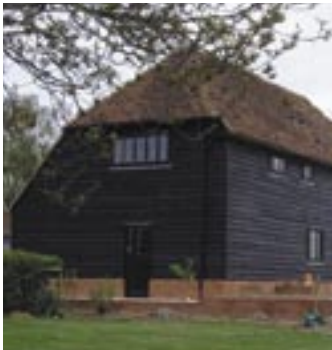
Country barn-style house Orlestone Oak supplied, constructed and erected the timber frame for this traditional barn-style house.
