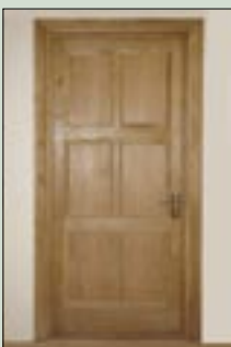
INo7: Heavy oak six panelled door and frame.
