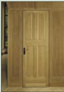
INo13: Understair panelled oak door.
