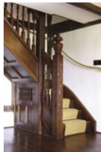
A traditional hand-carved oak staircase, stained and waxed for an antique finish.
