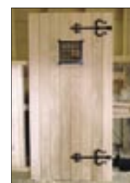
EX10: Framed ledge and brace door with cast iron grill over vision panel.
