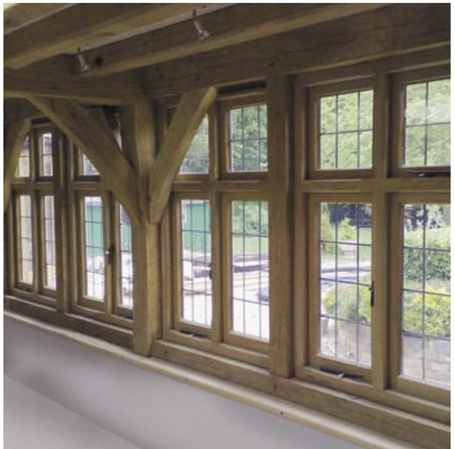
Solid oak windows manufactured and fitted to complement a period property.
