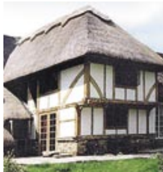
Oak framed extension This extension was designed and constructed by Orlestone Oak. The new frame design used the same traditional construction techniques as the original building.
