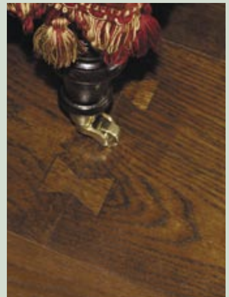
Detail of dovetail jointing on Jacobean stained and waxed flooring.
