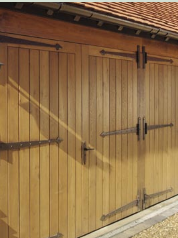
EX22: Framed, ledge and brace double oak doorsets fitted into a garage complex including strap hinges supplied by Orlestone Oak.
