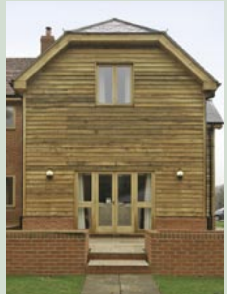
Orlestone Oak supplied many oak components for this new-build house. This included oak soffit boards, oak fascia panels, oak barge boards, oak feather-edged weatherboard and glazed French door screen.
