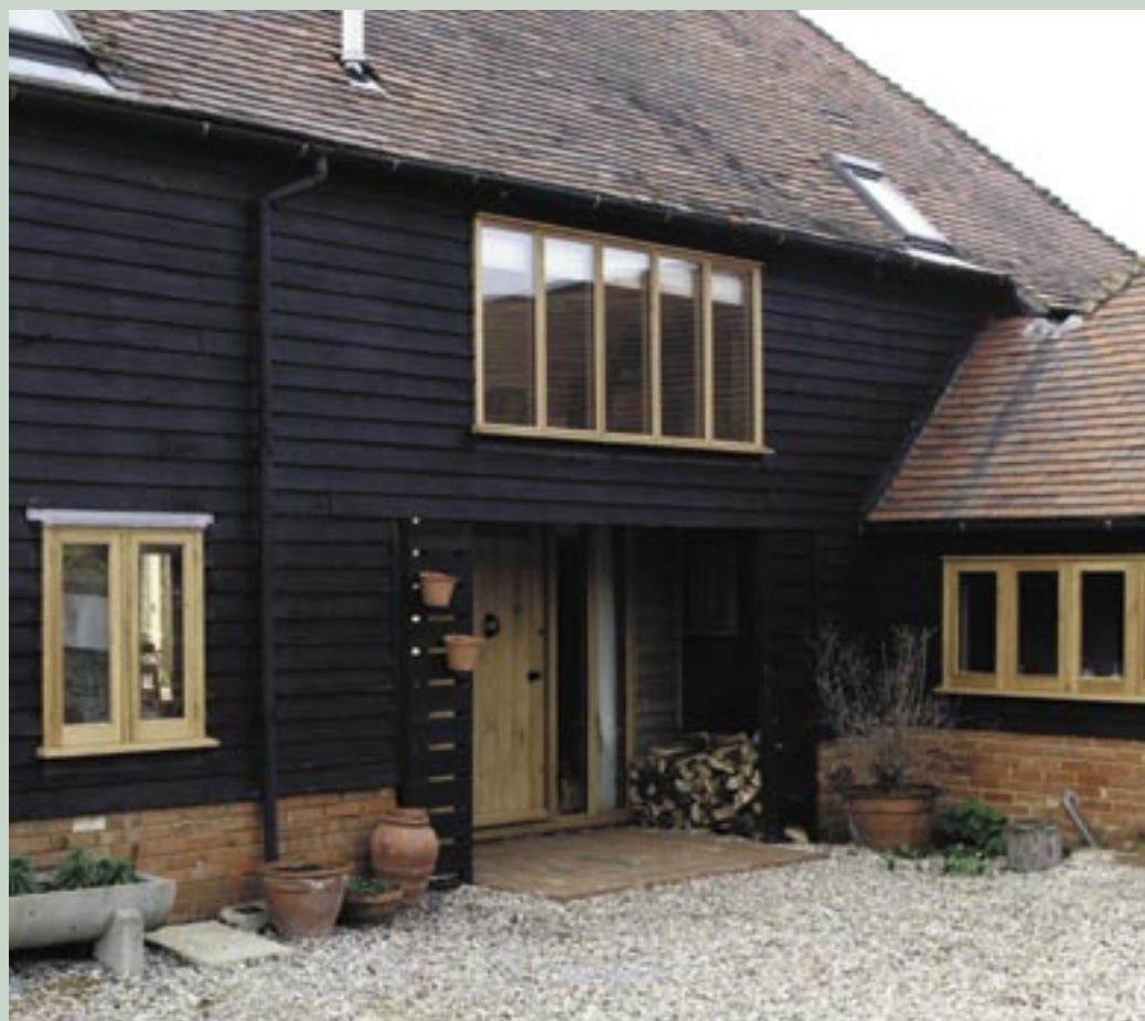
Orlestone's ovolo oak framed window profile (above) in a period property. Windows were supplied with leaded glass and complementary ironmongery.
