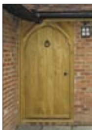
EX02: Gothic arch-topped oak door with heavy 4 inch frame.
