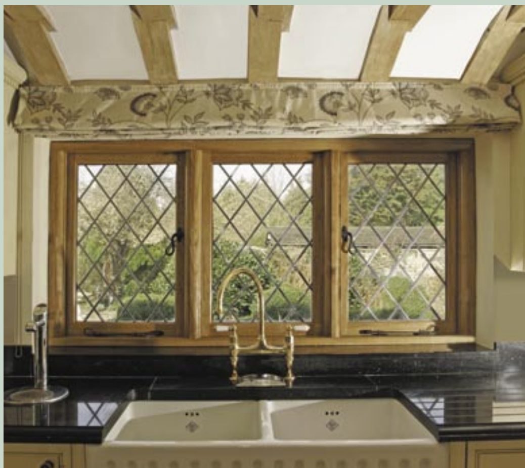
Orlestone's ovolo oak framed window profile (above) in a period property. Windows were supplied with leaded glass and complementary ironmongery.
