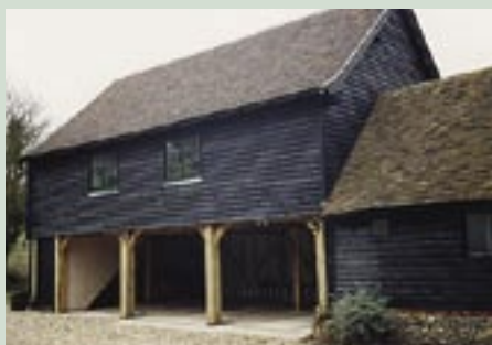
Two-storey garage/hobby room
