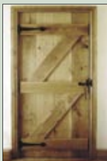
INo2: Standard ledge and brace internal oak door with traditional ironmongery.
