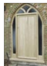
EX15: Gothic arched oak door frame with decorative features and panelled oak door.
