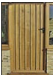
EX03: External oak door with vertical fillets as the main feature.
