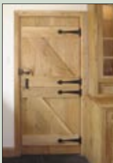
INo3: Split oak stable door, ledge and brace design.
