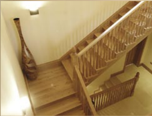
A traditional hand-carved oak staircase, stained and waxed for an antique finish.
