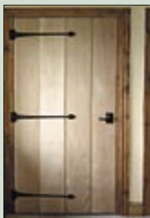
INo1: Ledge and brace oak door. To achieve a higher fire rating 32mm thick ledge and braces were used.
