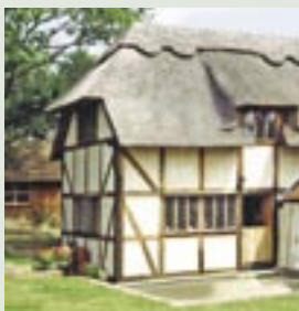
A traditional oak framed house, extended using the same design and building methods as the original construction.
