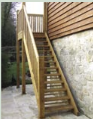
External oak staircase for access to upper floor of oast house.
