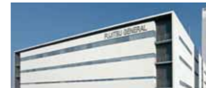
JAPAN Head Office R&D Center And 60m Height Difference Testing Tower
