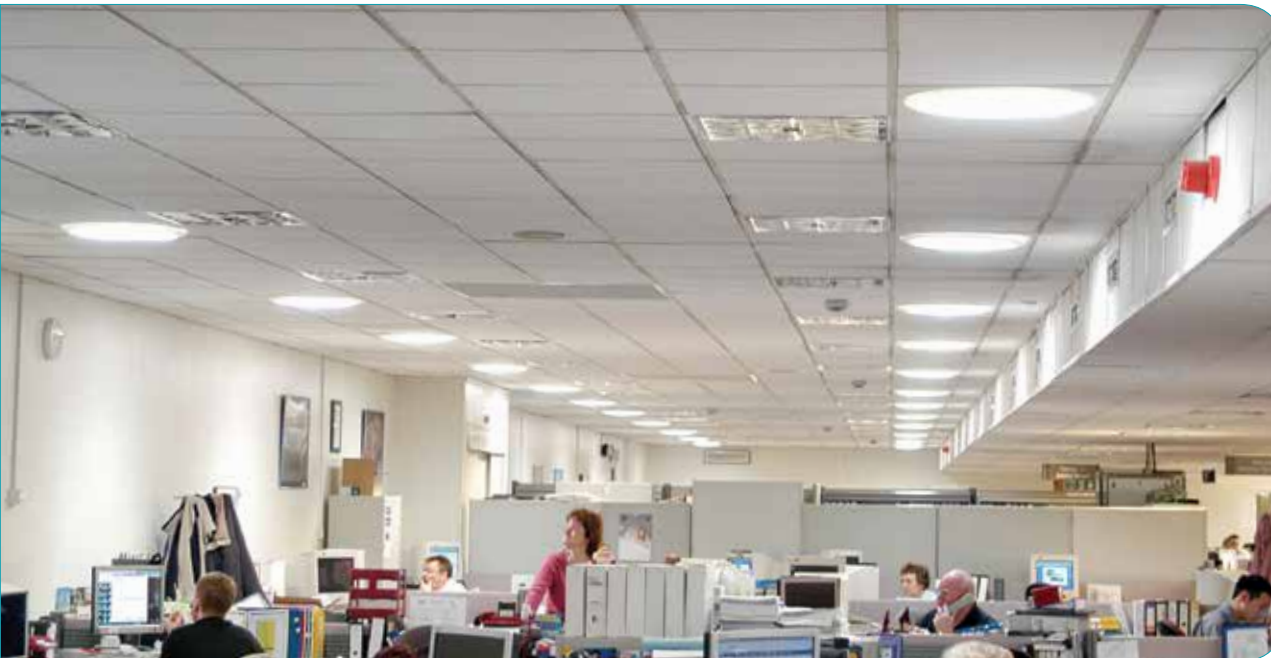
Above: Internal view of WINDCATCHER and SUNPIPE systems installed at the Daimler Chrysler offices in Milton Keynes
