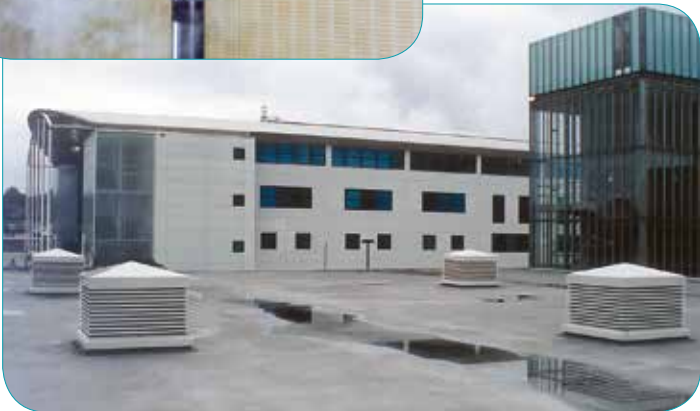
Below: WINDCATCHER systems installed on flat roof of old central mainframe computer building
