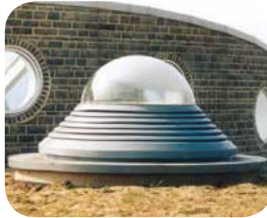
Natures World, Middlesbrough where a 1500mm dia SUNPIPE system is installed
