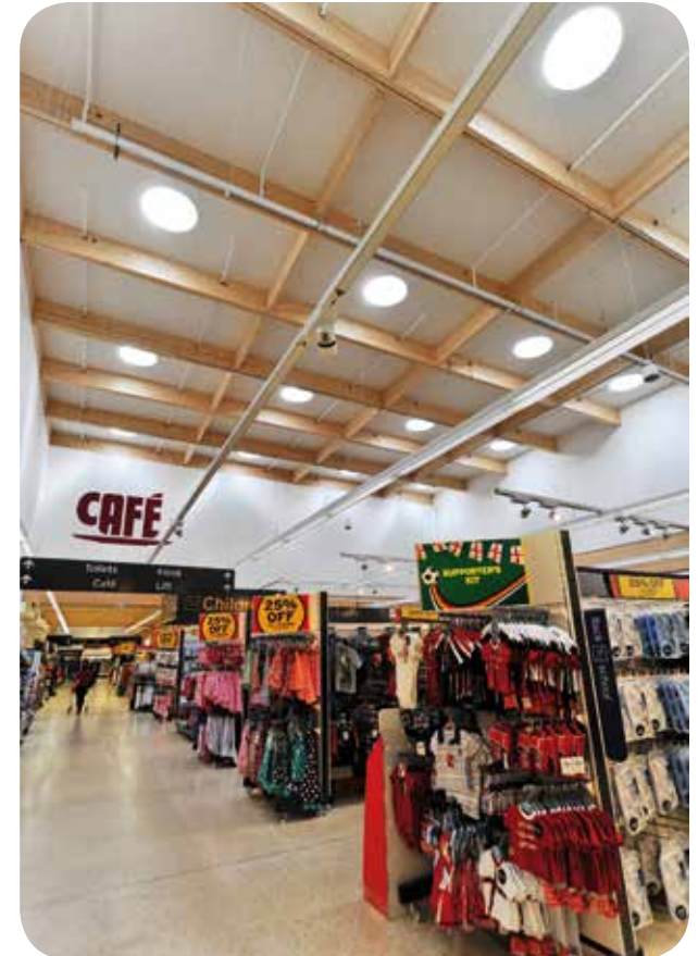
Sainsbury's, Durham - 1000mm diameter SUNPIPE natural daylight systems were used to light the double height sales area
