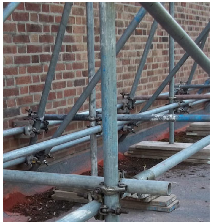
Cripple Bracket Scaffold System, RAF Station, Norfolk
