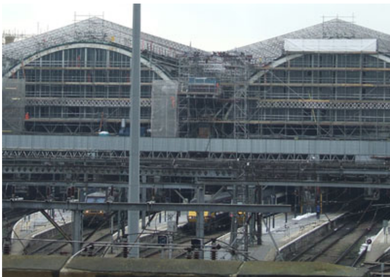
Northern Façade Scaffold, Kings Cross Station Refurbishment
