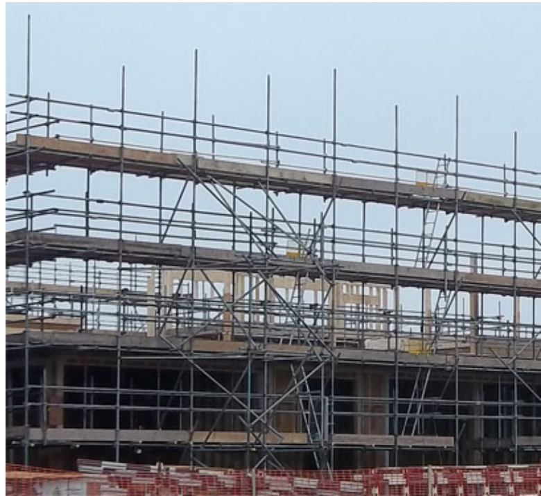
Free standing Scaffolding, New School, Wolverhampton
