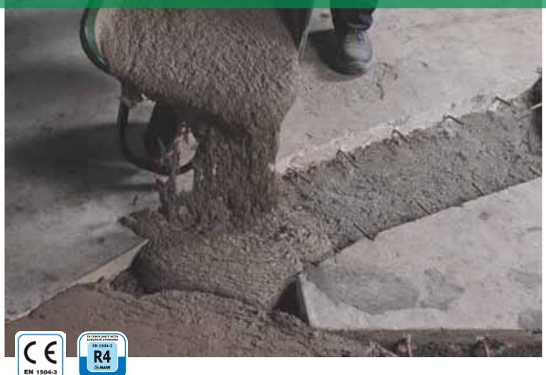
Castable rapid-setting and hardening, controlled-shrinkage, high-ductility mortar used in conjunction with metallic fibres (Fibres R38). Suitable for application down to -5°C.
