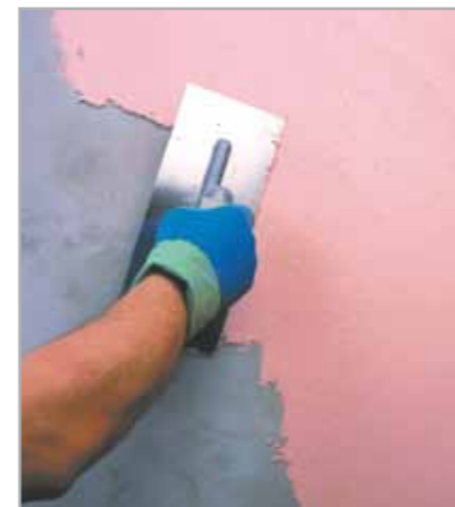
Fig. 5.18 – Apply the finishing layer of render
