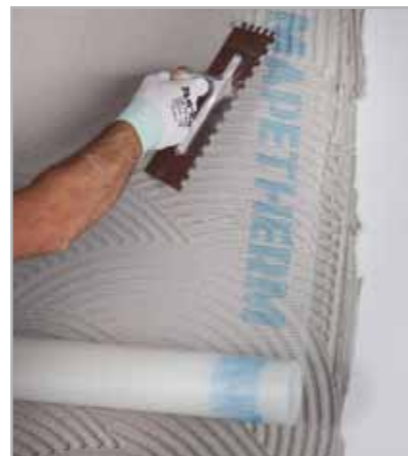
Fig. 5.16 – Lay on MAPETHERM NET
