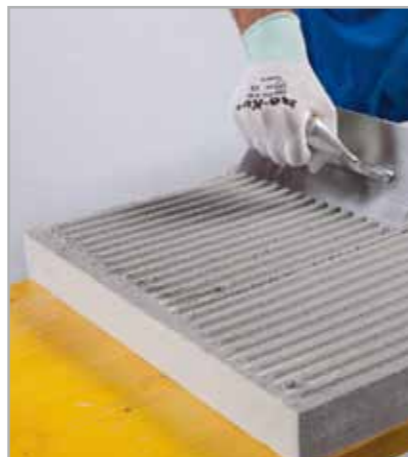
Fig. 5.8 – Spread an even layer of adhesive on the back of the insulating panel
