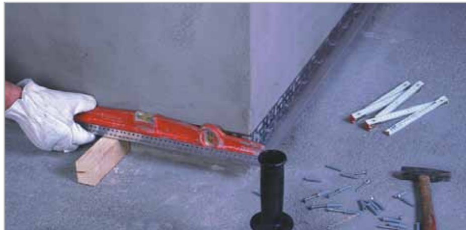
Fig. 5.6 – Position the support profiles: make sure they are horizontal using a spirit level
