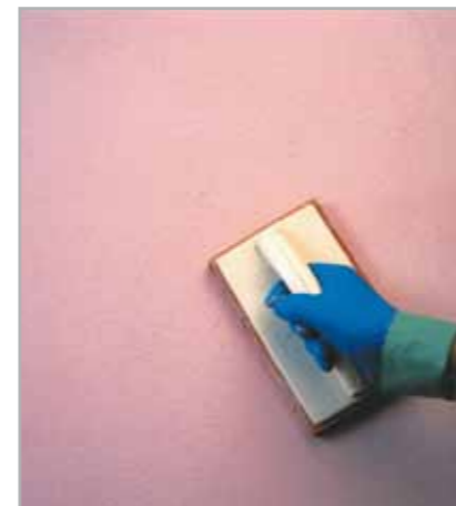
Fig. 5.19 – Finish off the surface of the render with a sponge float
