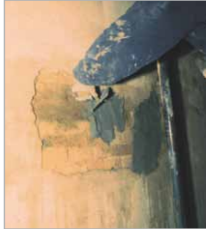
Fig. 5.5 – Rebuild the loose render with NIVOPLAN+PLANICRETE
