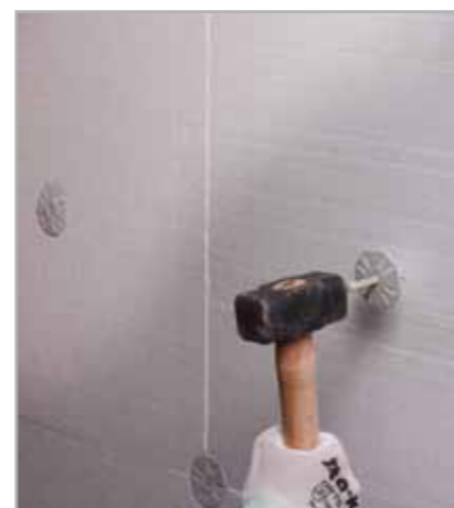
Fig. 5.13 – Insert the plugs
