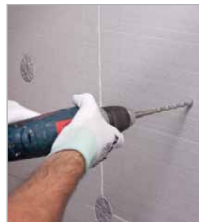
Fig. 5.12 – Drill holes for the plugs
