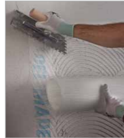
Fig. 5.17 – Overlap the edges of the net by at least 10 cm
