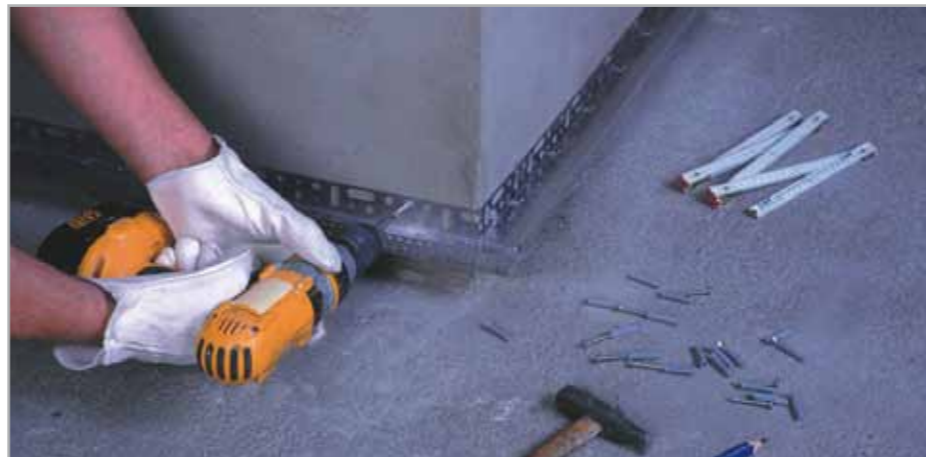
Fig. 5.7 – Fasten the support profiles in place using expansion plugs
