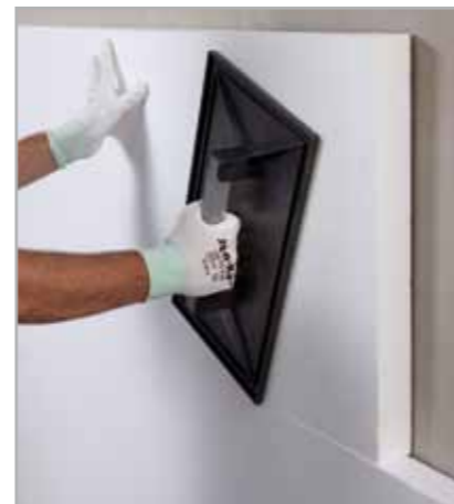
Fig. 5.11 – Press down the panel with a float
