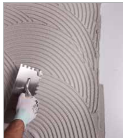
Fig. 5.15 – Apply the first coat of the smoothing and levelling layer
