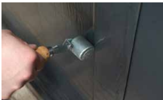
Use a roller to firmly press the membranes onto the substrate.
