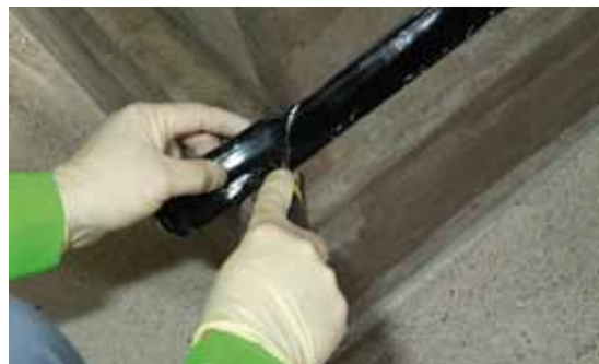
Fillets can be made of either KÖSTER Repair Mortar or alternatively with the cold self-adhesive KÖSTER KSK Triangular Ribbon.
