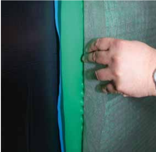
KÖSTER SD Sheet 3-400 protects the waterproofing and provides a drainage for residual water.
