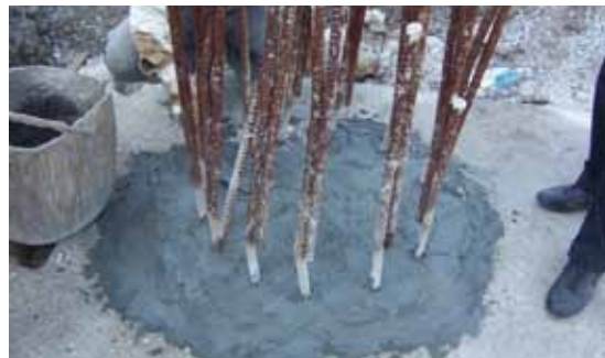
Installing a fillet and smoothing the area with KÖSTER Repair Mortar
