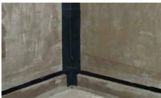
After that, the membrane is applied to inside and outside corners.
