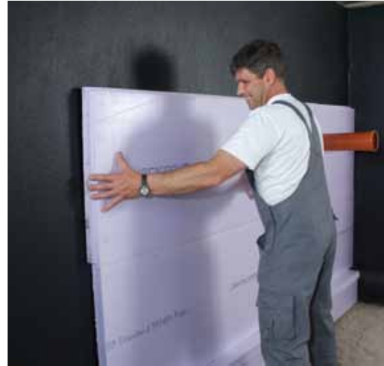
XPS boards spot bonded with KÖSTER Deuxan®
