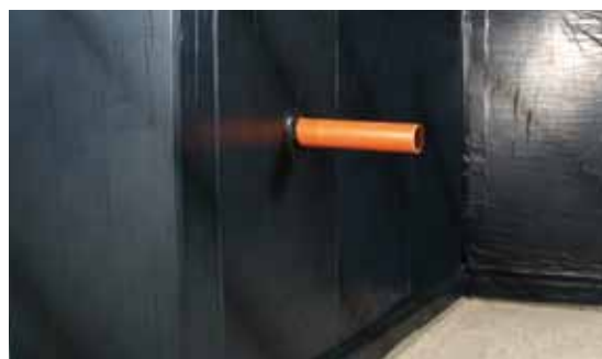
Finished waterproofing with KÖSTER KSK
