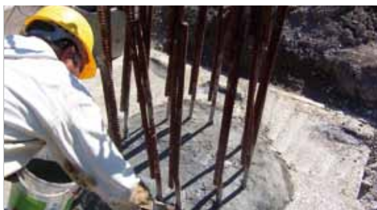
Waterproofing of the pile head with KÖSTER NB 1 Grey
