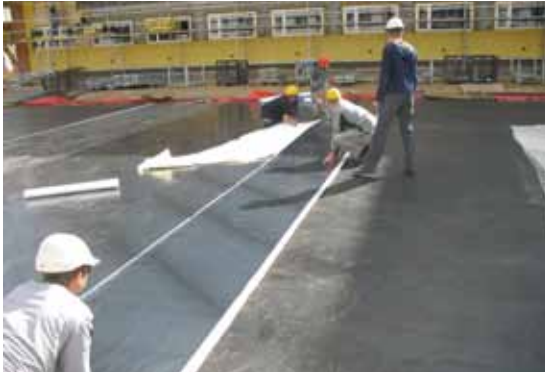
Waterproofing with KÖSTER KSK Membranes
