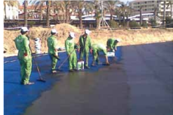
Waterproofing with KÖSTER Deuxan®
