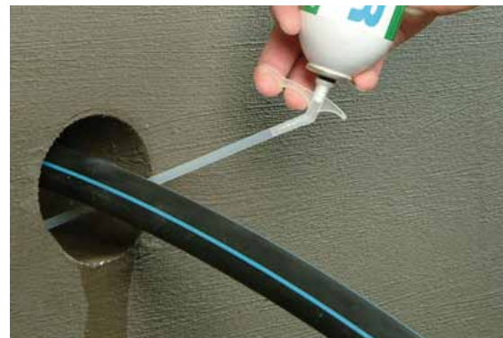
A PU-Foam is injected in order to have a backing for the KÖSTER KB-Flex 200.
