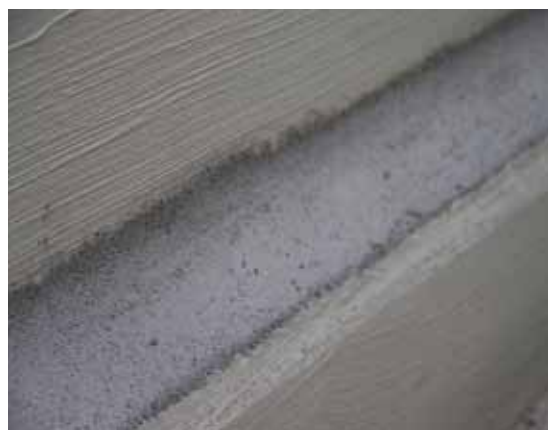
A concave fillet in the wall-floor junction with KÖSTER Repair Mortar
