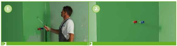
KÖSTER BD 50 is applied to the area using a roller or a brush. Application of waterproofings is always done in at least 2 coats. Consumption per coat is approx. 0.5 to 0.6 kg/m² leading to a total consumption of approx. 1.1 kg/m². Waiting time between coats is at least 3 hours.
