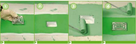
Position the KÖSTER Floor Sleeve over the floor drain on which it is applied. Cut a hole of the shape of the opening of the inside area of the floor drain into the KÖSTER BD Floor Sleeve. The hole should be smaller than the drain so that it overlaps approx. 3 mm. Apply a covering coat of KÖSTER BD 50 to the area around the floor drain where the KÖSTER BD Floor Sleeve is going to be installed.
