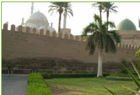
Example for rising damp
