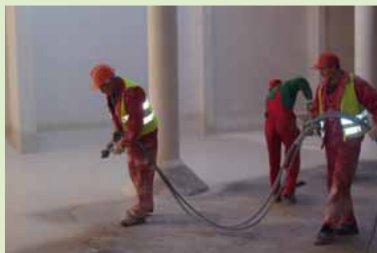
Drinking water tank, Tarnów, Poland
