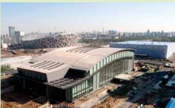
Olympic hall, Beijing, China
