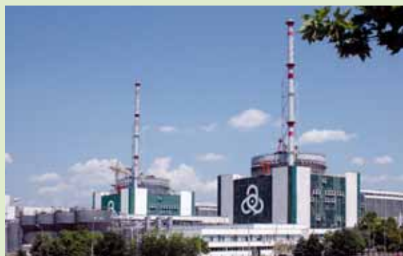
Nuclear power station, Sofia, Bulgaria
