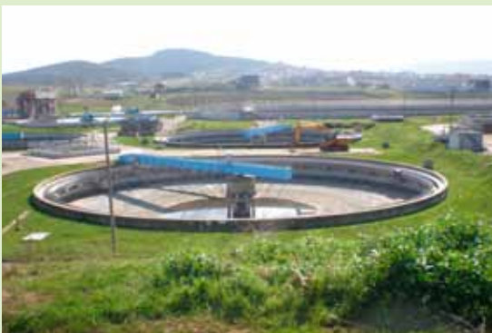
Sewage treatment plant, Istanbul, Turkey
