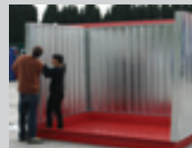
3. FIT PANELS TO THE EXPANDACHEM BASE
