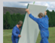
4. SLIDE IN THE WALL, DOOR + WINDOW PANELS
