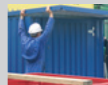
5. LIFT ON AND FIX THE ROOF
