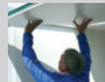
6. SLIDE IN THE CEILING PANELS
