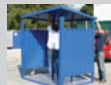
6. LIFT ON AND FIX THE ROOF
