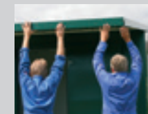
7. FIT THE OUTER ROOF SKIN
