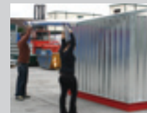
5. LIFT ON AND FIX THE ROOF
