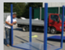
3. FIT CORNER POSTS TO THE BASE
