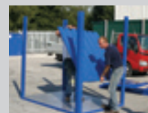
4. INSERT THE SIDE WALL PANELS
