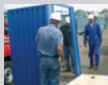
3. FIT PANELS TO THE EXPANDASTORE BASE
