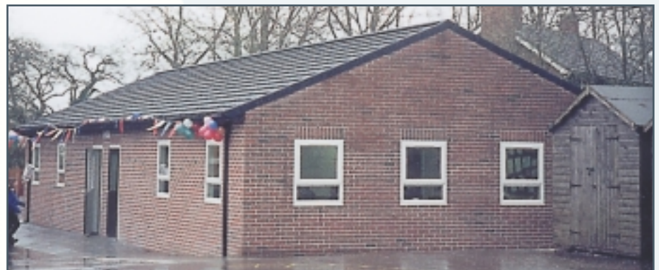
Modular building with pitched roof and brick cladding
