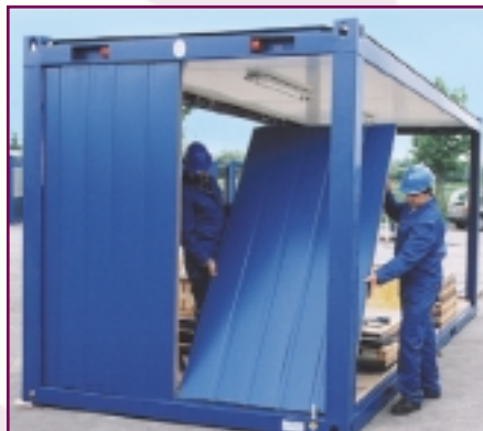
The TransPAK structure can be changed at any time after installation by removing wall panels
