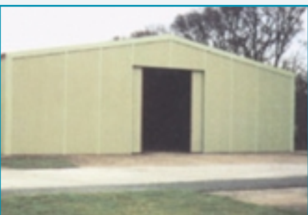
Industrial building with box profile plastic coated steel cladding
