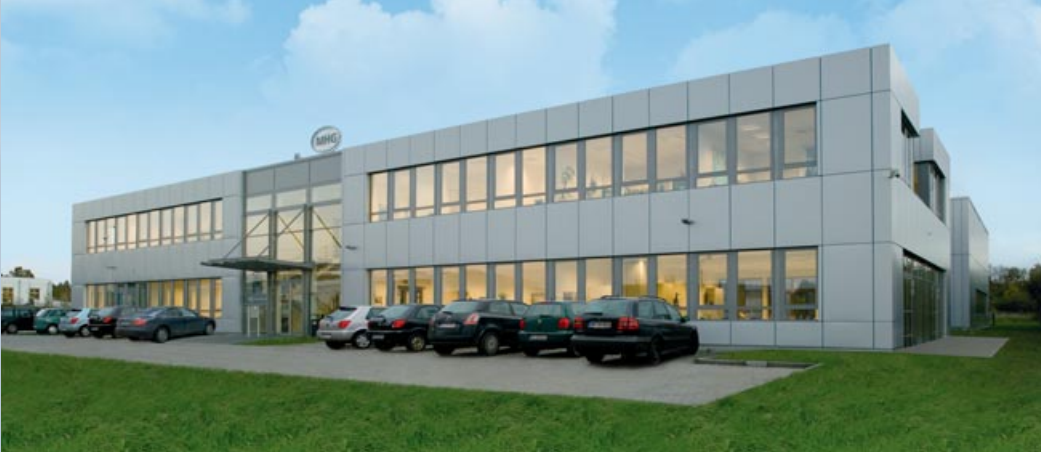
MHG's head offices are in Buchholz near Hamburg.
