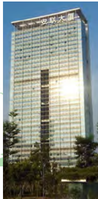
GELEC Office, Shenzhen, China
