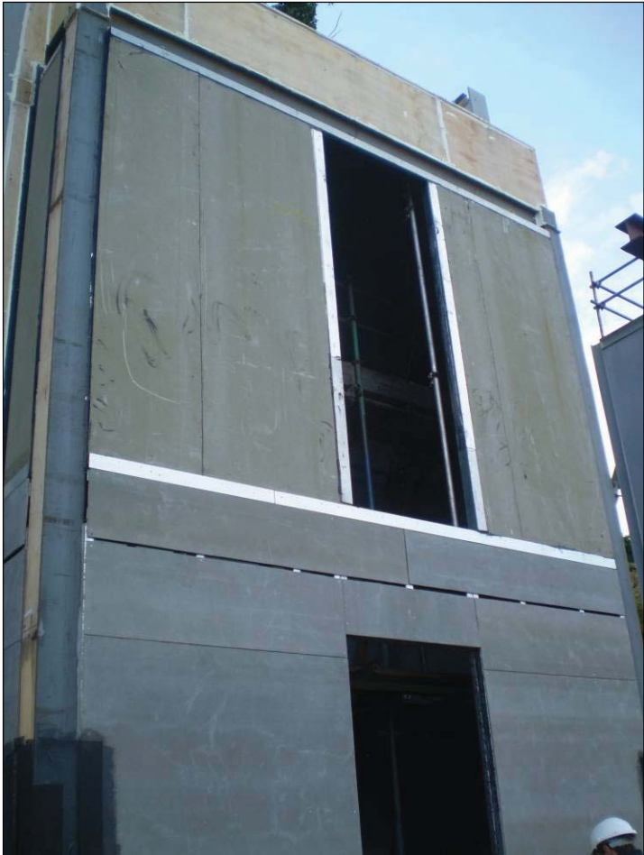
TEST SAMPLE DURING CONSTRUCTION
