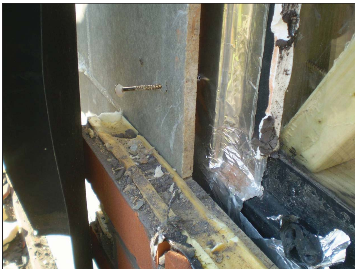
BOTTOM CORNER DRAIN AT PERIMETER OF WINDOW OPENING
