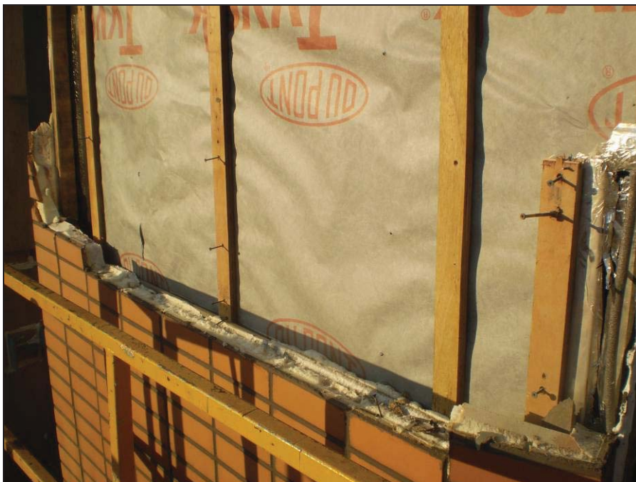
UPPER GEBRIK PANELS REMOVED
