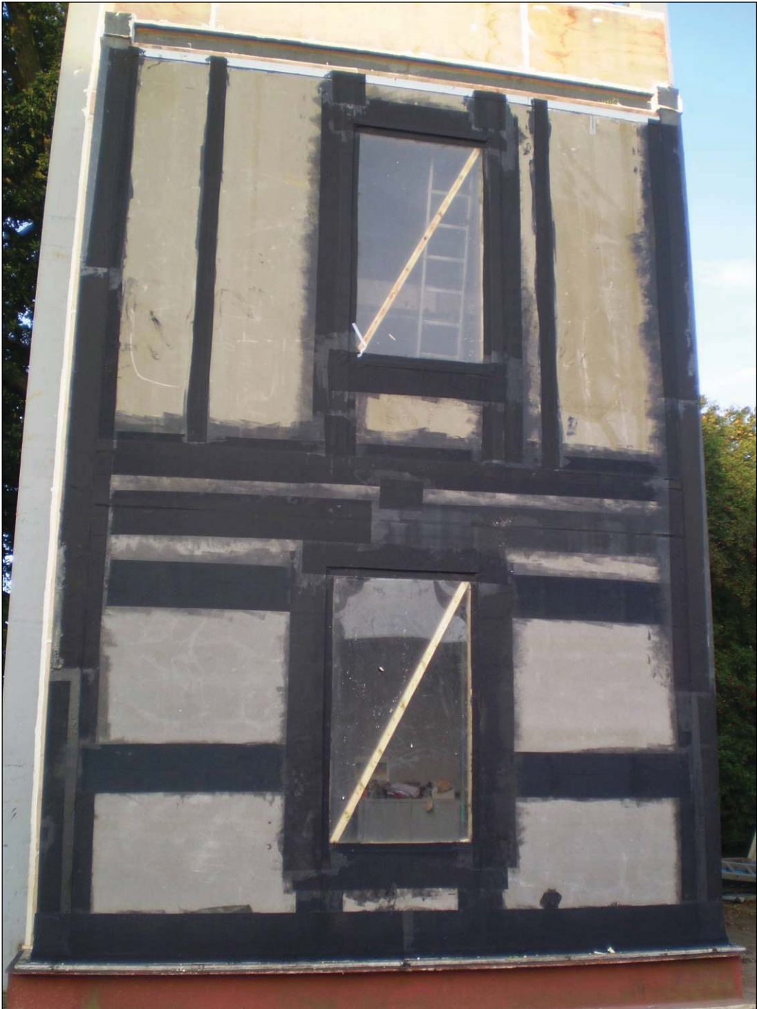
TEST SAMPLE DURING CONSTRUCTION
