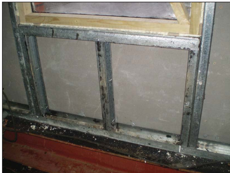
INTERNAL VIEW BENEATH LOWER WINDOW OPENING
