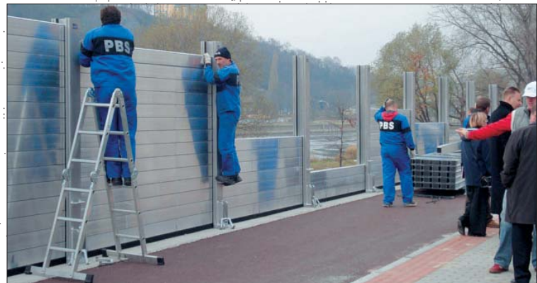
Insertion of Dam Beams
