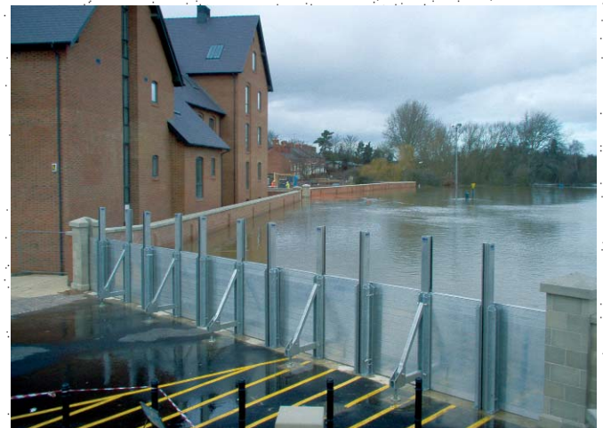
Demflood system creating a new flood storage area
