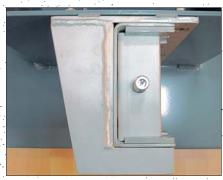
Assembly in front of the channel with dowels in case of tensile and pressure load. The end posts are placed in front of the channel with spread anchors. Shear connectors can be used alternatively for attachment. The end posts are mounted on base plates. Gusset plates are installed between the end posts and the base plate to meet static requirements.
