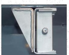
Assembly in front of the channel pressure load only towards the building. The end posts are placed in front of the channel with spread anchors. Shear connectors can be used alternatively for attachment.
