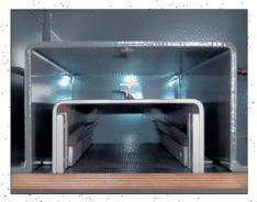
**Assembly in first concrete.** The end posts are attached directly to the formwork and embedded in the concrete.
