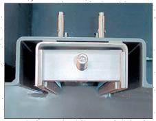
Assembly in recess. The end posts are dowelled into the construction recess. Then the front side is pared and cast in with a non-shrinking mortar.
