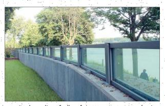
It was crucial for the glass wall sections to be as long as possible to reduce the number of support posts so as not to obstruct the views, but at the same time the sections had to be robust enough to withstand the heavy loads. With this in mind high performance laminated safety glass was used combined with slim yet exceptionally strong frames, this allowed spans of 2 m in length.
