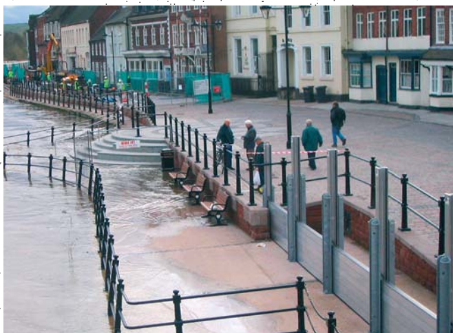
Firstly, full height barrier system installed
