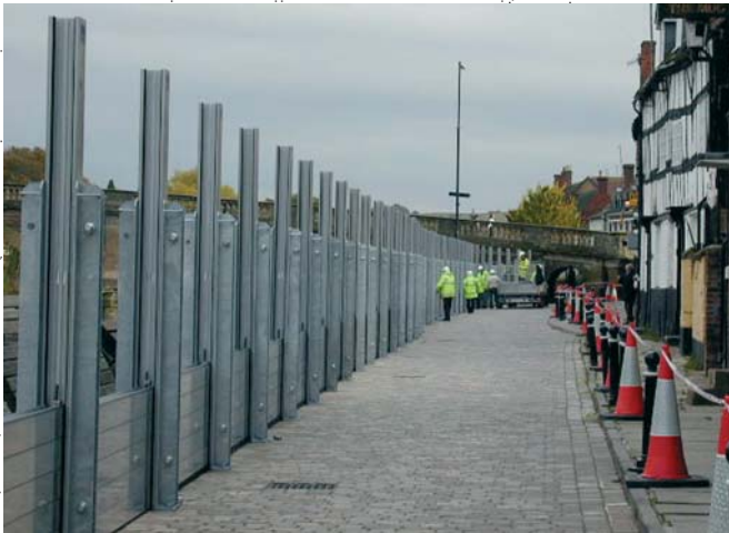
Full system erection at minimum defence height
