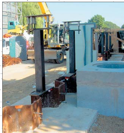
Assembly on sheet piling with cantilever for height compensation
