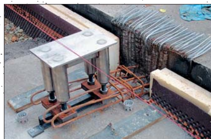
Assembly on subbase
