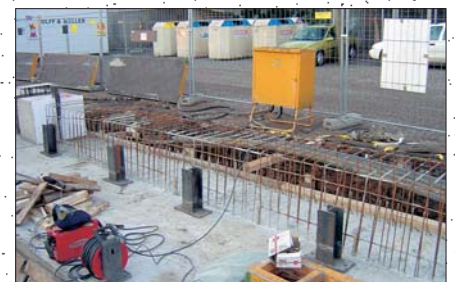
Assembly on subbase with cantilever for height compensation
