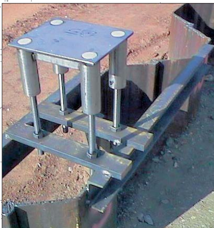
Assembly on sheet piling
