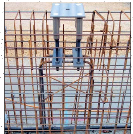
Assembly on construction joint with binder made of concrete reinforcement steel
