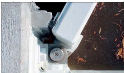
Connection at abutment and seal
