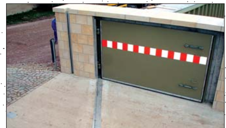
Bottom sill acts as horizontal wing support in passages
