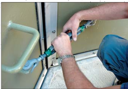
Impermeability is achieved by tensioning
