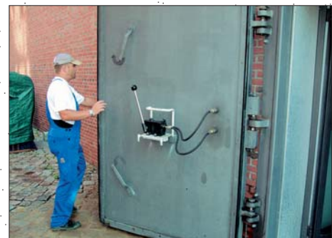
Mobile hydraulic manual pump for lifting/lowering the door wing into the door hinges
