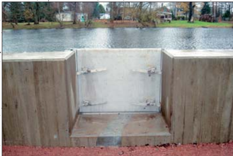
Contact pressure is achieved using four brackets
